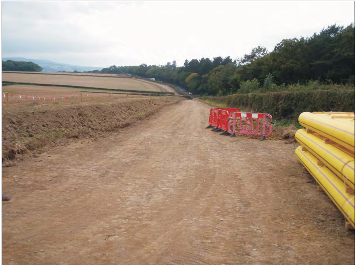
Plate 1: General view of route, looking northwest from Plot 4
