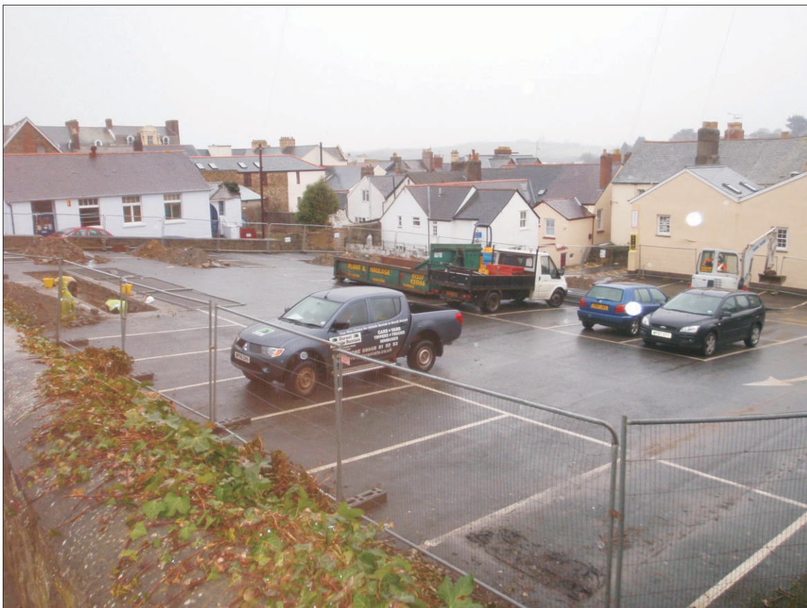
Plate 2: Excavations in Bridge Street car park. Looking northeast
