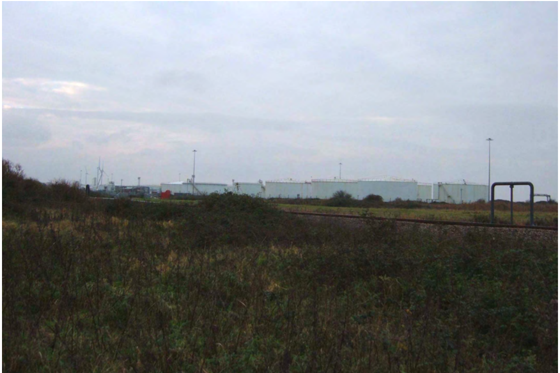
Plate 1: View to the south-west showing railway line and fuel storage depot within Avonmouth Port Authority land. The proposed cable trench route is adjacent to the railway line
