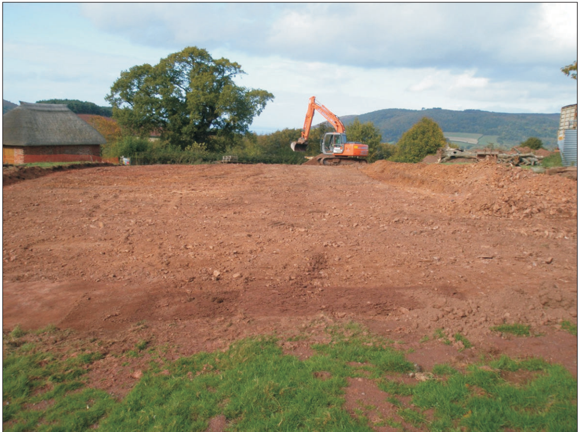
Plate 4: Soil stripping for the new barn, view to west
