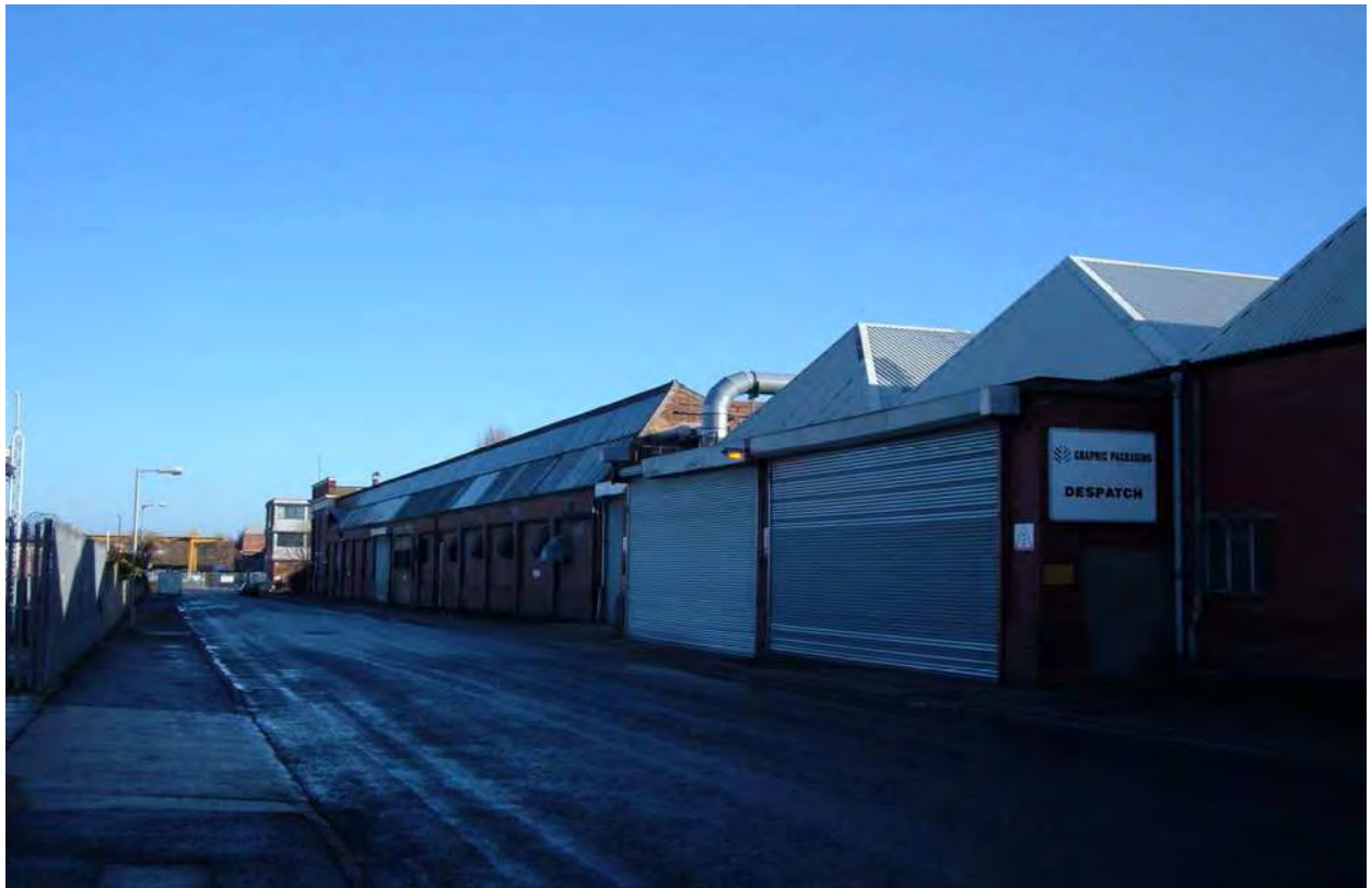
Plate 3: View to NE along Goodneston Road
