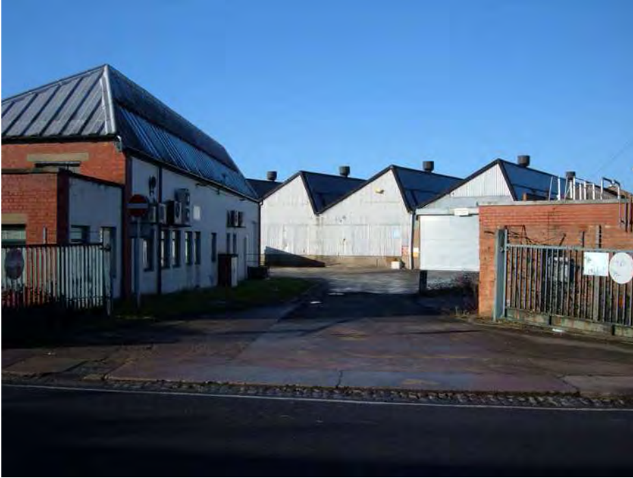
Plate 6: Site entrance onto Enfield Road. View to W
