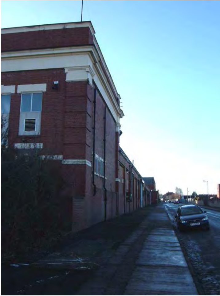
Plate 2: Detail of NW corner pavilion; view to SW along Goodneston Road
