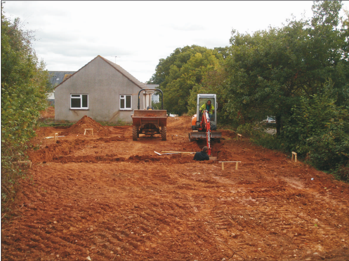
Plate 1 General view of site, facing southeast
