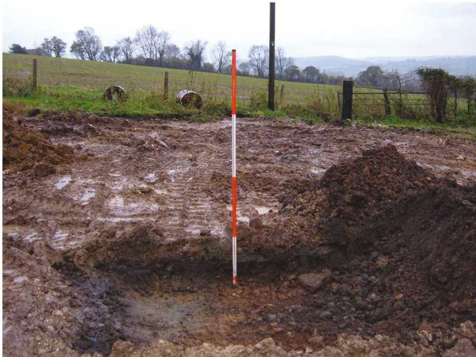
Plate 4: Trench 3 (view to the south). 2m scale
