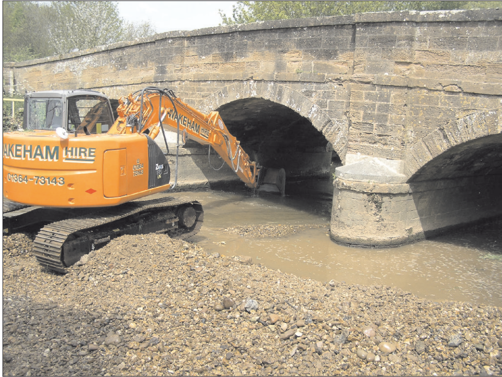
Plate 1: Dredging beneath Arch B, view to northwest
