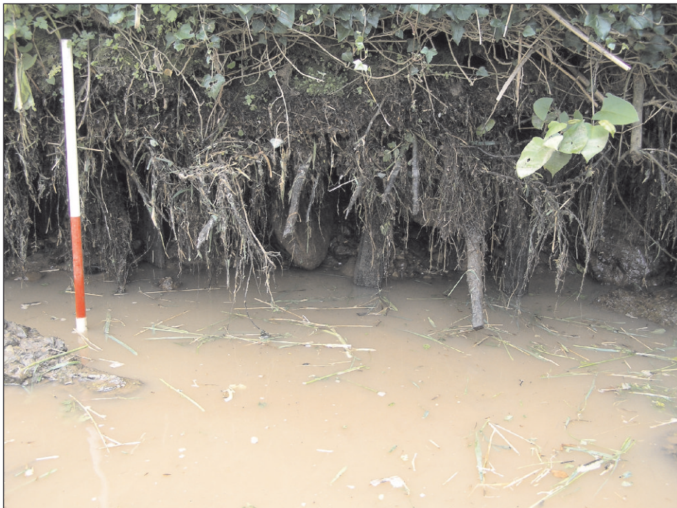
Plate 2: In situ timber stakes on east bank, view to east (exposed scale 1m)
