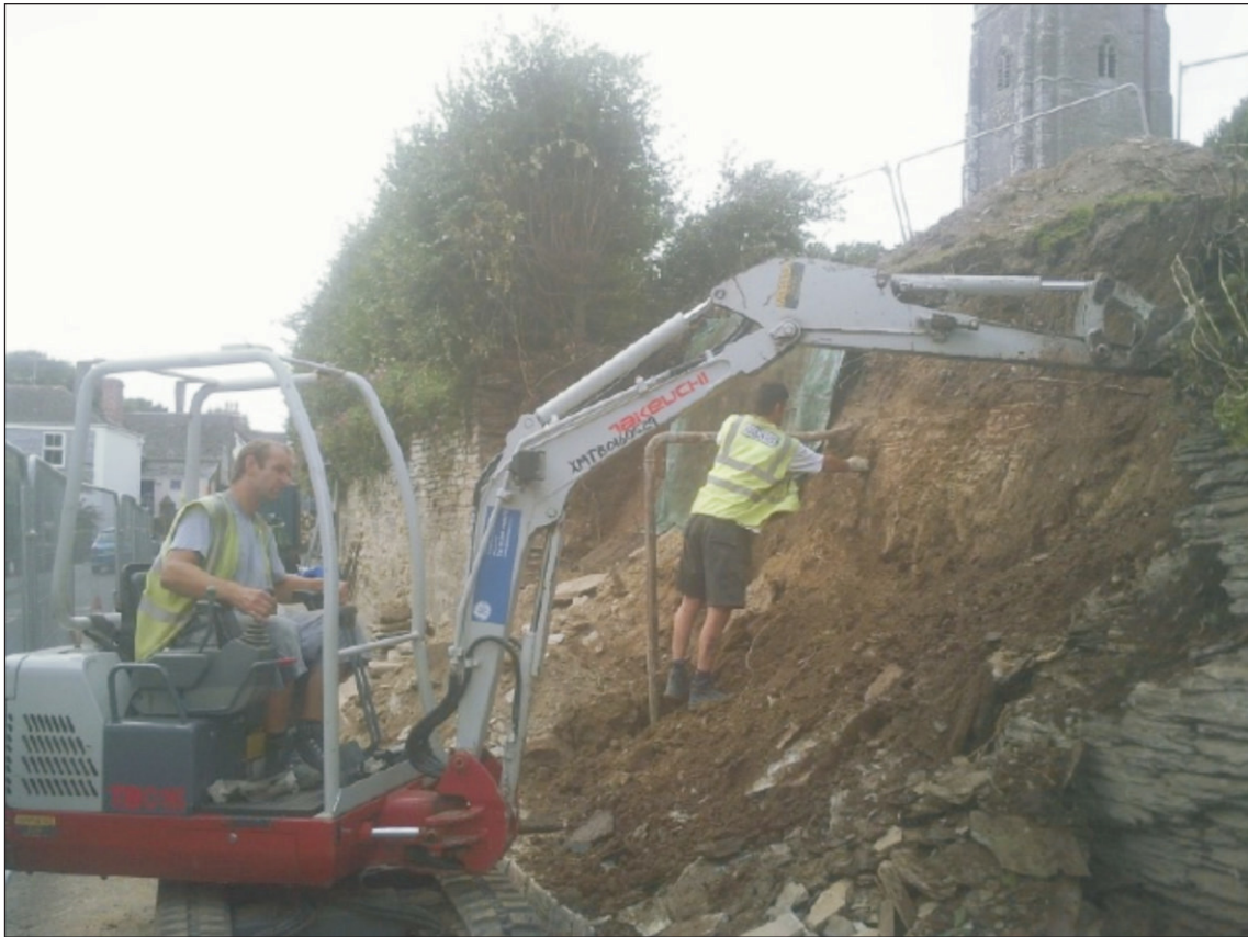
Plate 5: Works to remove wall, view to northwest
