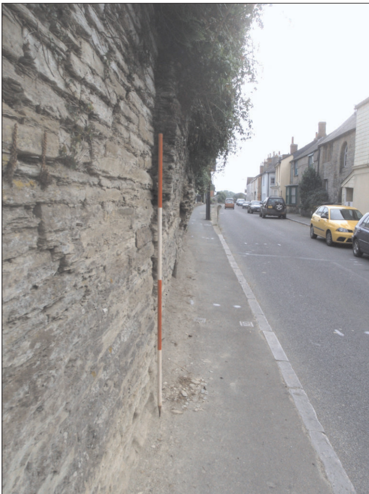
Plate 2: Detail of wall, view to east (Scale 2m).
