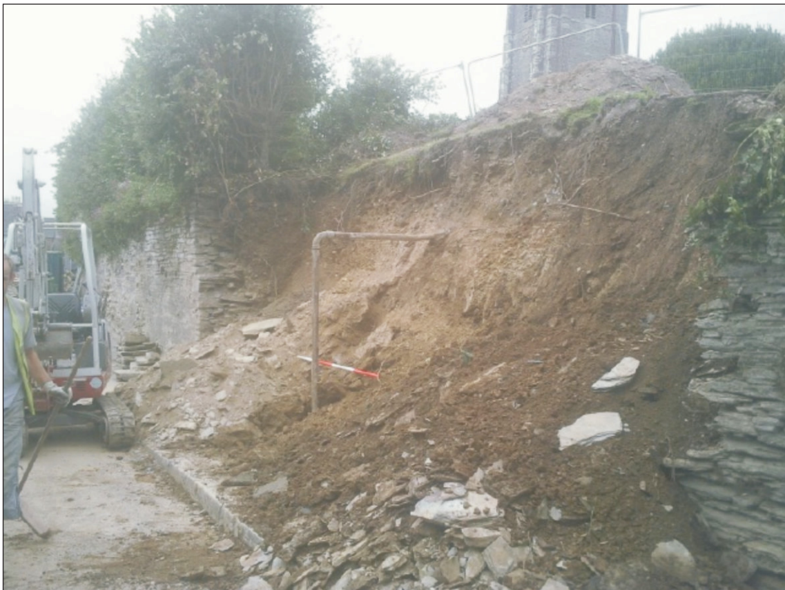
Plate 6: Exposed soil profile to rear of wall (Scale 2m)
