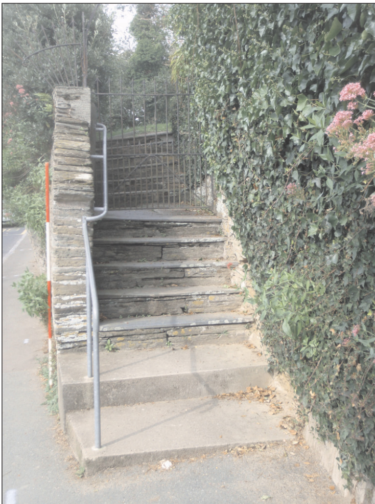
Plate 4: Steps at southeast corner of churchyard, view to west (Scale 2m)
