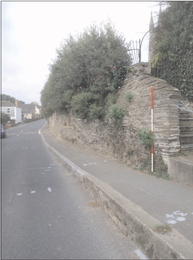
Plate 3: East end of wall and steps, view to west (Scale 2m)
