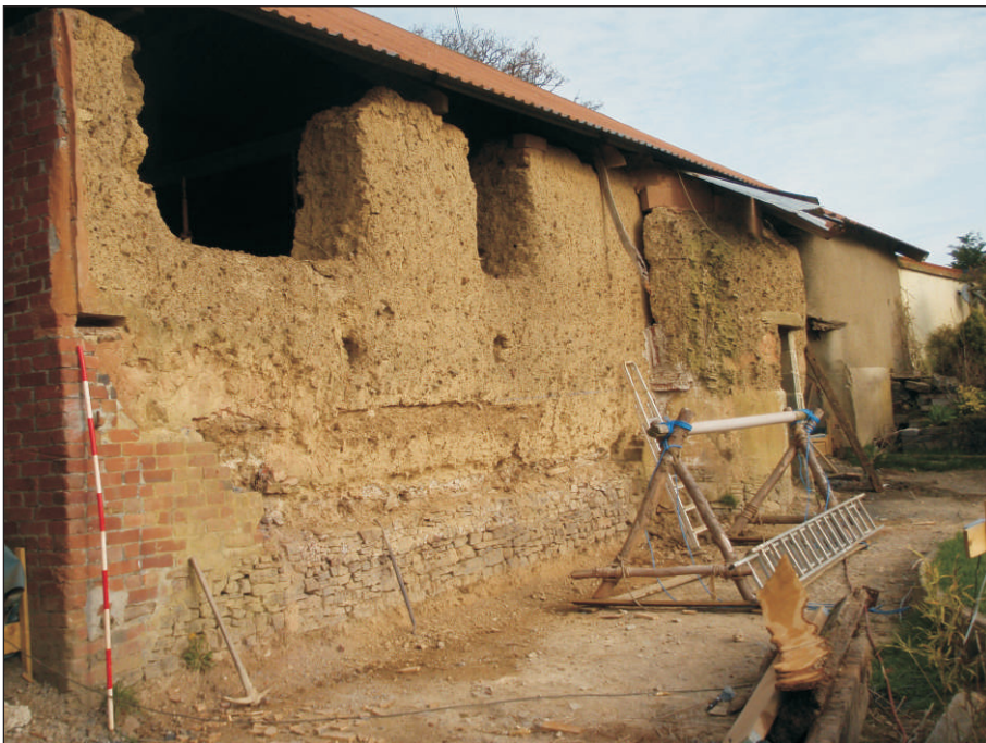
Plate 2. West elevation of barn, view to the northwest. (Scale 2m)
