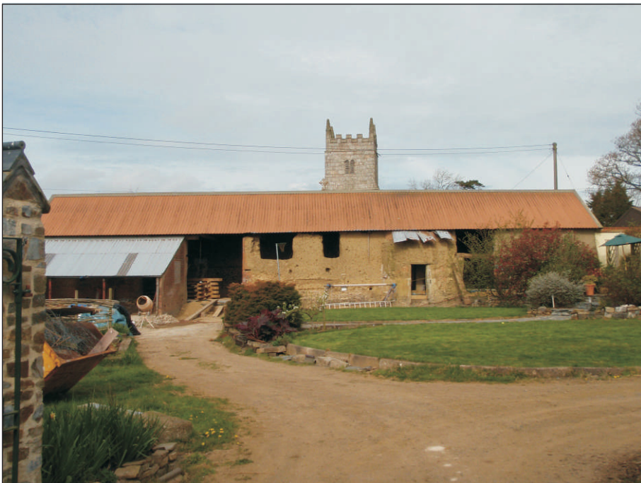
Plate 1. General view of the barn, looking to the west
