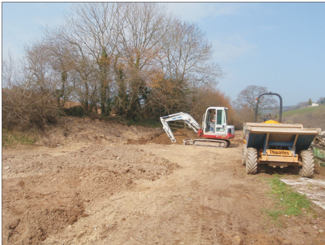
Plate 1. General view of site, looking north
