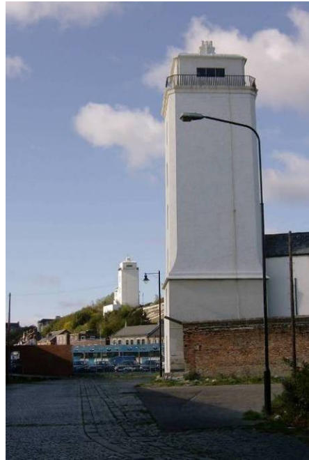
Figure 7.14 The ‘New’ High and Low Lights at North Shields (author)
