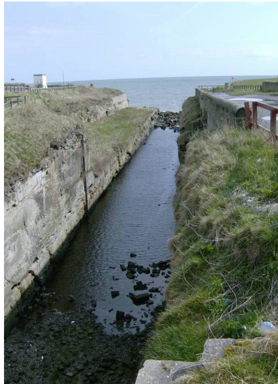
Figure 7.9 The rock-cut, artificial harbour at Seaton Sluice (author)
