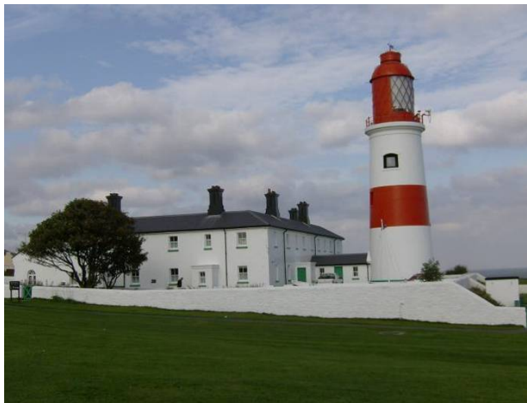
Figure 7.11 The Grade II* Lighthouse at Souter Point (author)
