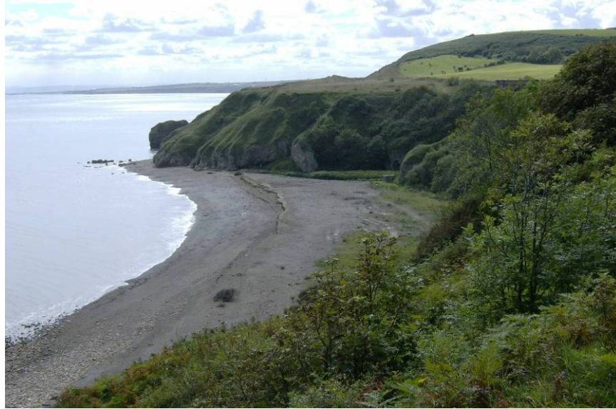
Figure 7.2 Eroding colliery waste at Hawthorn Hive, County Durham (author)
