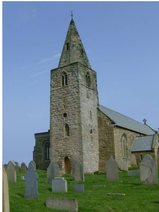
Figure 8.7 St Bartholomew's Church, Newbiggin (author)
