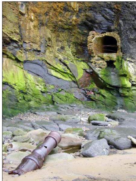
NERCZA2_0065: GPS 24-25. Outfall Sewer
