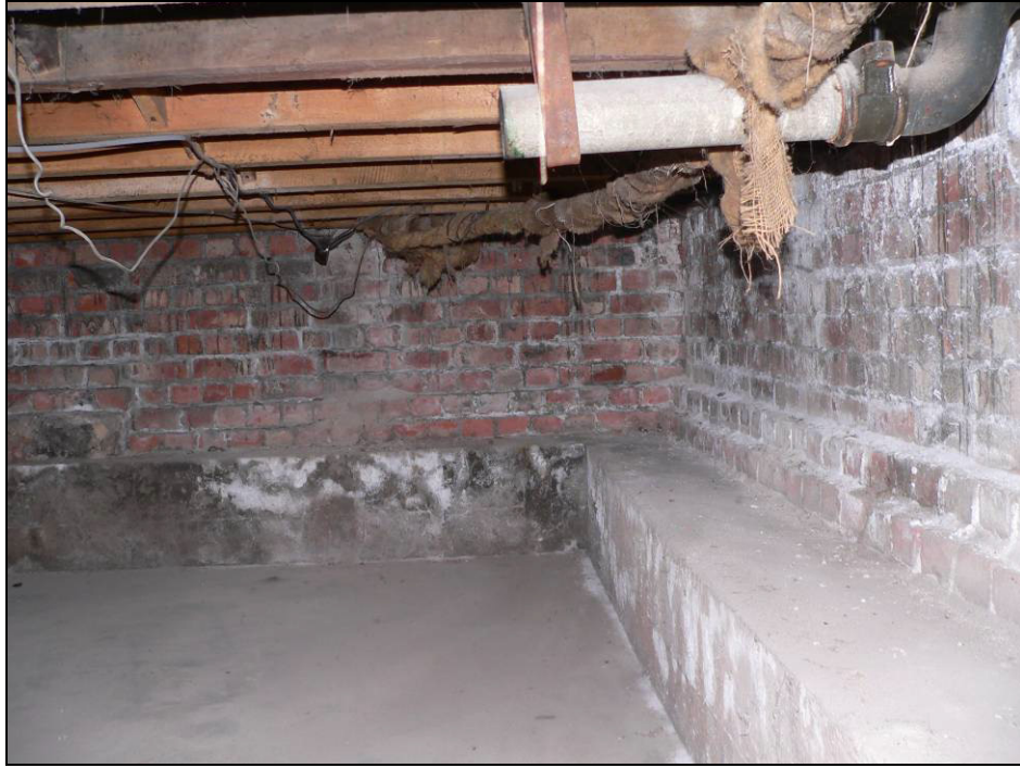
Fig 5.7.14 The basement level.
