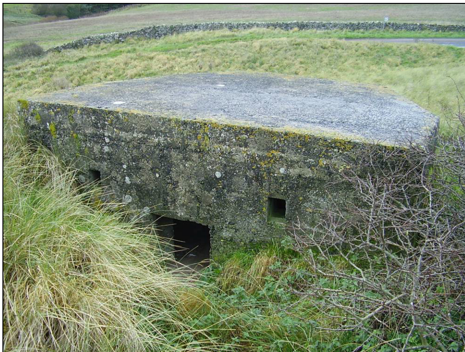
Fig 5.15.8 The rear entrance of the same pillbox.
