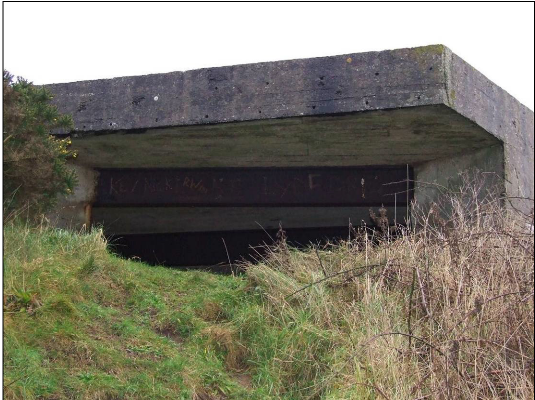
Fig 5.16.13 Budle battery (500), clearly demonstrating scale of construction.
