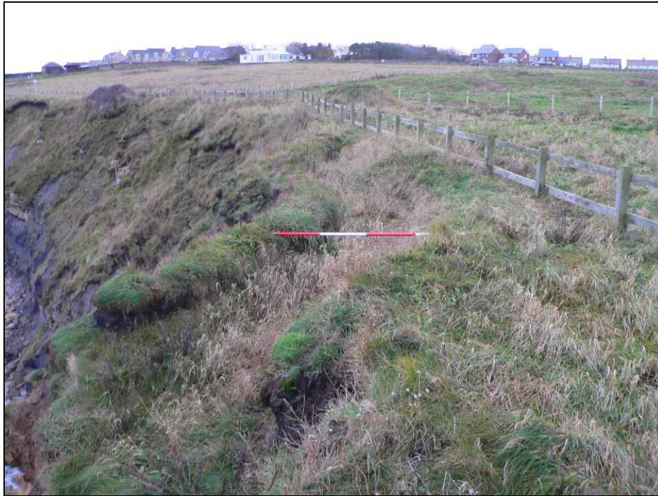
Fig 5.7.17 eroding trench (444) on the cliff edge with Fort House in the background.
