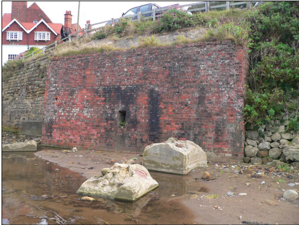
Figure 5.2.10 Anti-tank blocks in Sandsend beck beneath the remains of a former brick-built railway viaduct.
