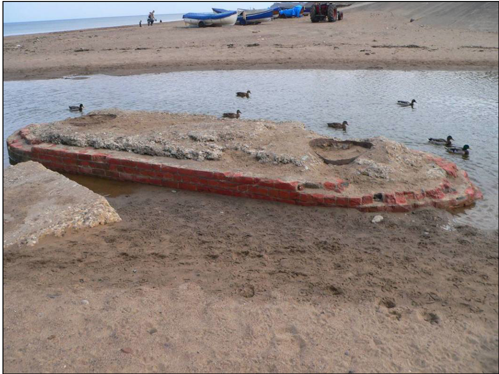
Figure 5.2.8 Pier base for a now removed 19 th century railway viaduct at Sandsend Beck looking south with an in situ WWII anti tank cube in the foreground.
