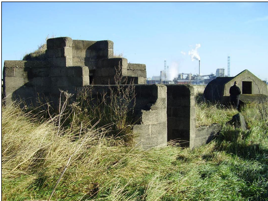
Fig 3.4.4 Generator house for bombing decoy with Stanton shelter in background.
