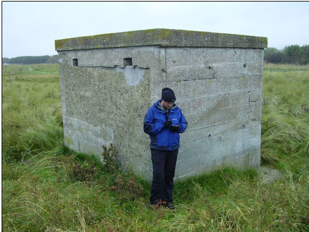
Fig 5.8.10 One of the observation posts. Note the large blocked entrance and aperture at the front, distinguishing it from a pillbox.
