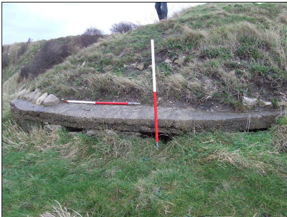
Fig 5.7.20 Circular pillbox (505) on Sandy Island, partially buried in sand.
