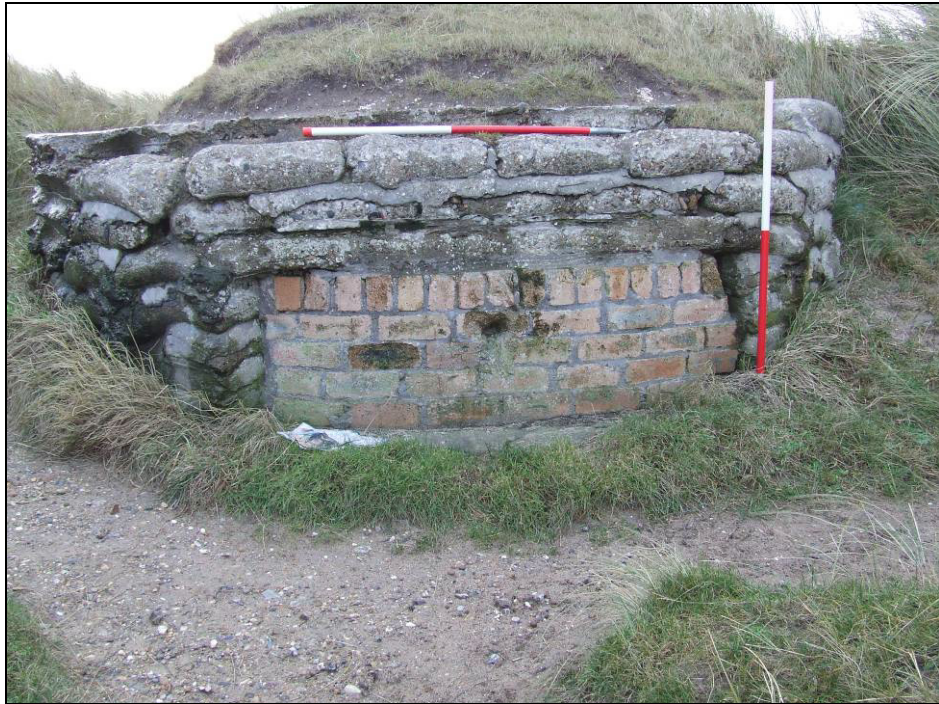
Fig 5.7.21 Circular pillbox (506) showing brick-blocked aperture.
