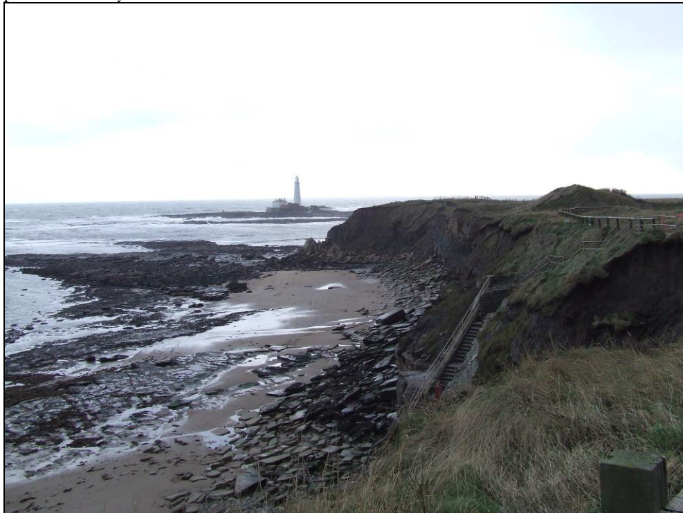
Fig 5.7.23 The eroding cliffs at Hartley with St Mary's Island and lighthouse in the background.
