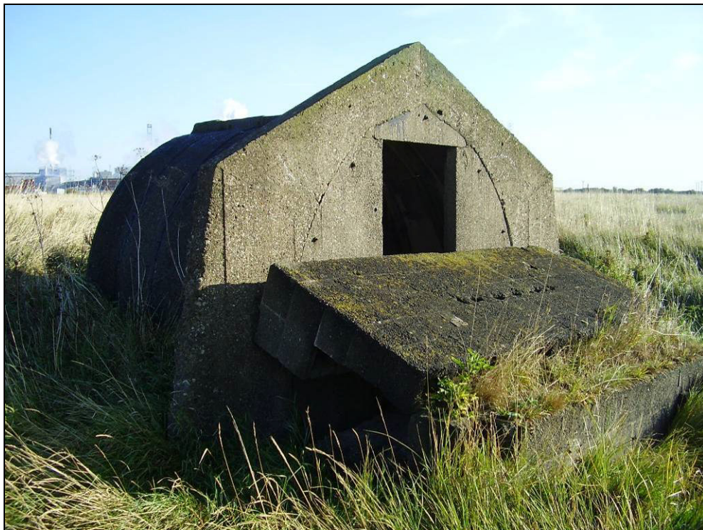
Fig 5.4.3 Stanton type air raid shelter at Greatham Creek, part of former bombing decoy.
