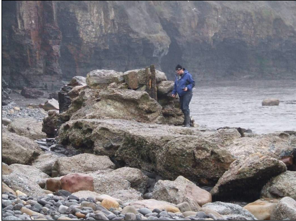
Figure 5.2.14 A rapidly eroding Alum pier at Sandsend that is exposed to direct wave action.
