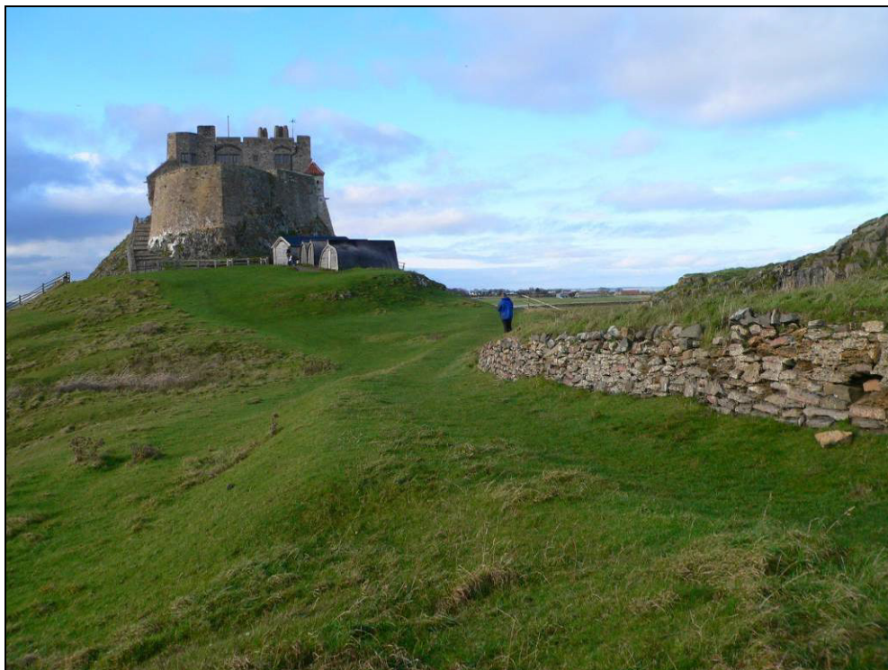
Fig 5.14.15 The stone built fire step, or loading bay and raised bank for the lime kilns.
