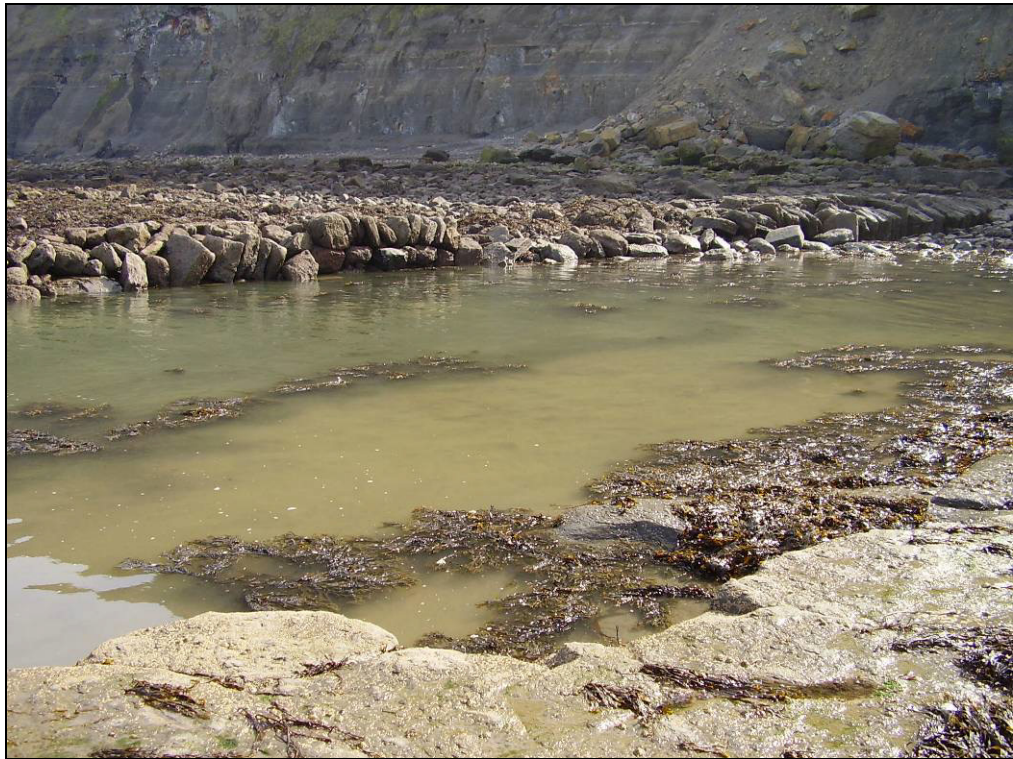
Fig 5.3.13 Surviving extent of stone alum pier at Loftus
