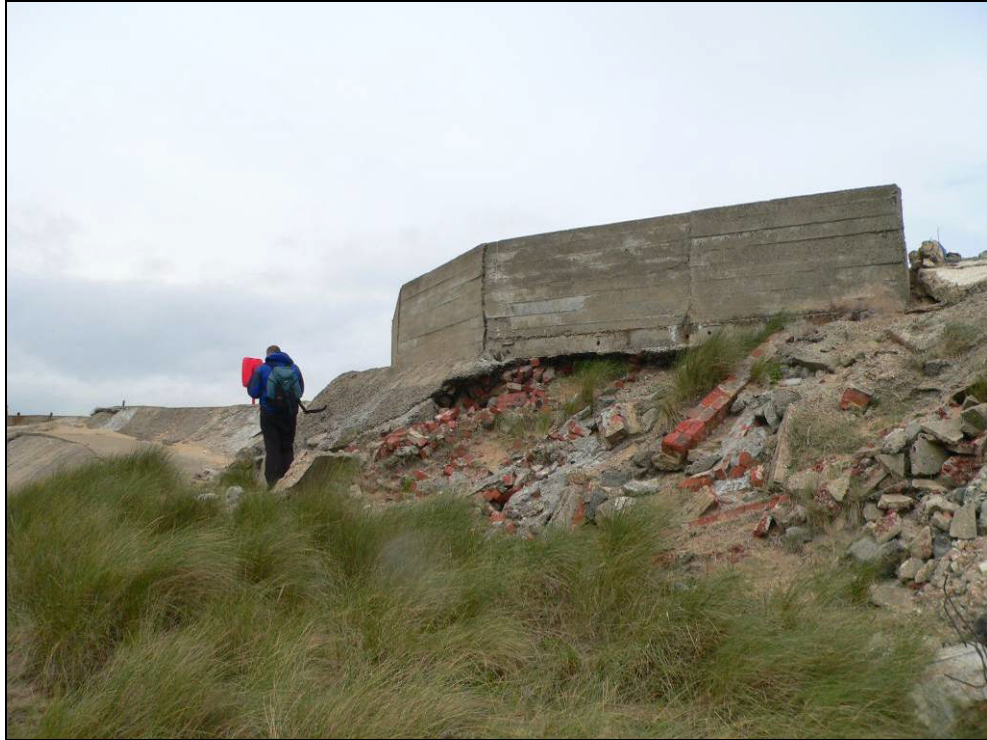
Fig 5.4.10 The remains of pillboxes used to reinforce the North Gare pier
