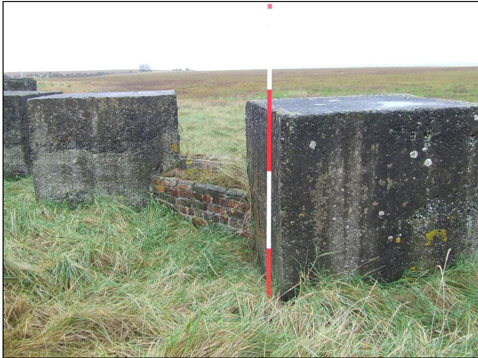
Fig 5.13.11 Anti-tank blocks at Fenham with a small brick built shooting butt or defensive wall clearly visible.
