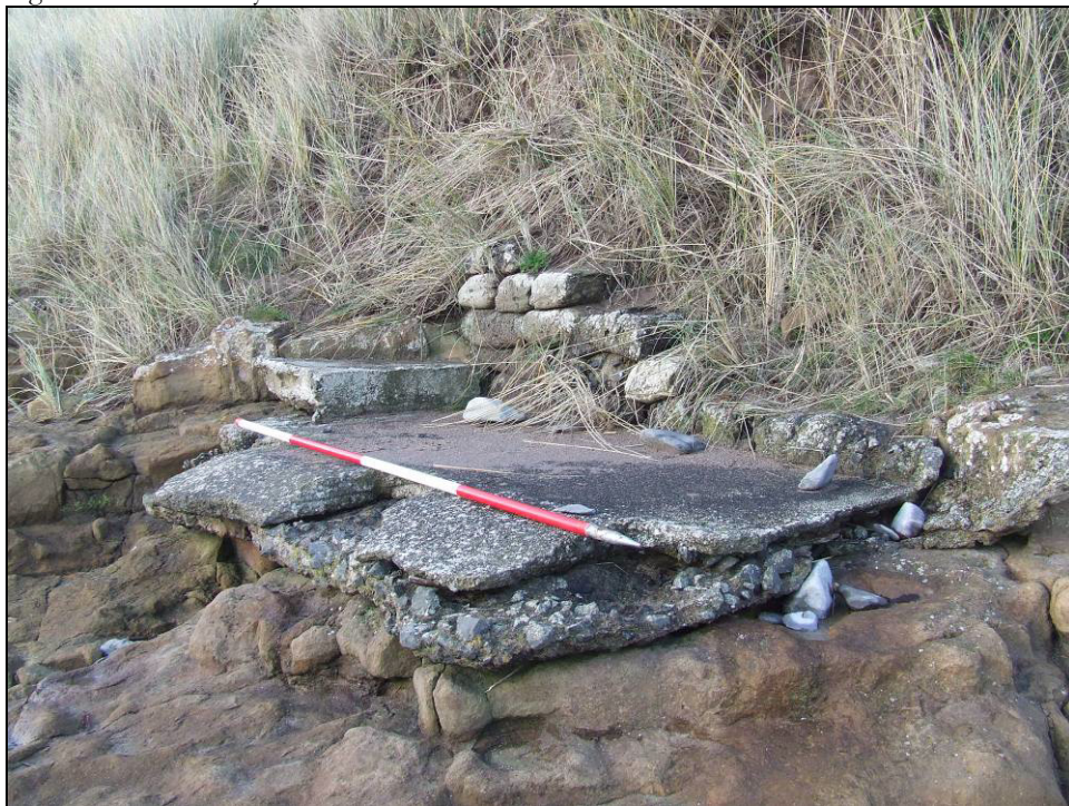
Fig 5.12.9 eroding concrete structure built utilising concrete sandbags, possibly of Second World War date.
