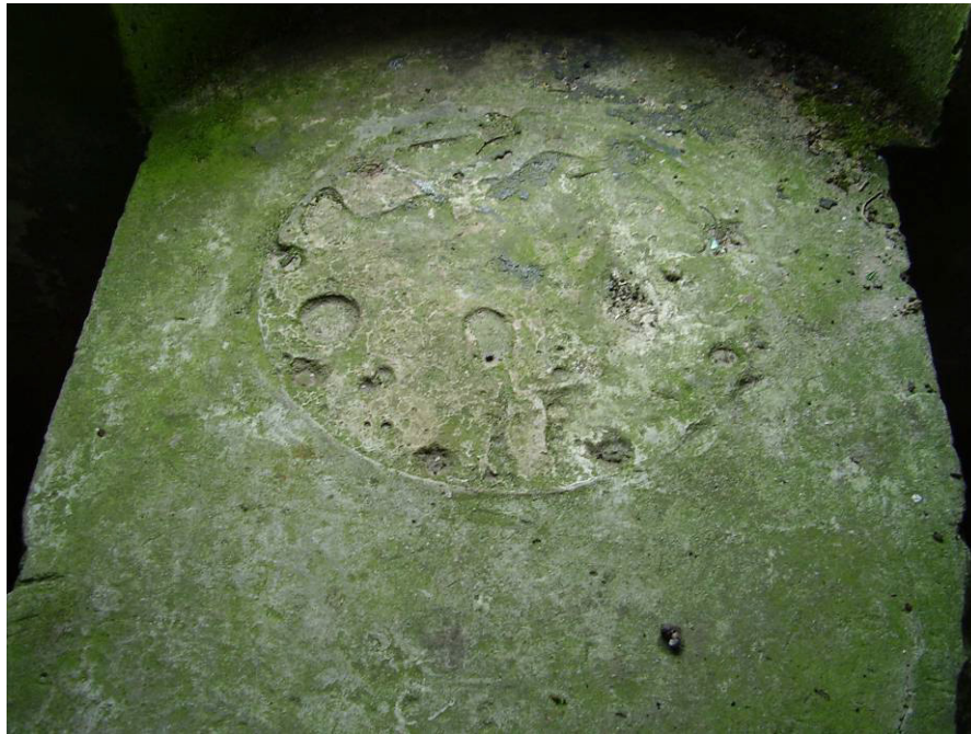
Fig 5.15.11 The concrete mounting for a 6 inch gun which would have been overlain by a metal mounting for the gun to swivel on.
