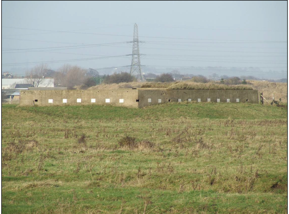
Fig 5.4.12 'Fortlet' 152 overlooking Greatham Creek made up of two large section posts.
