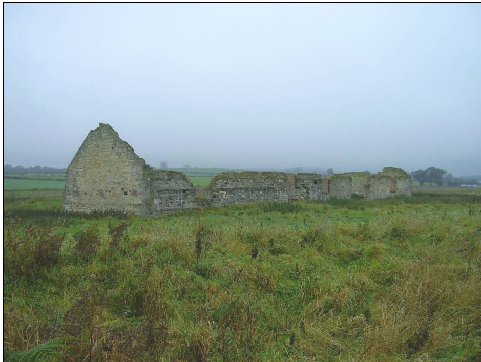
Fig 5.10.13 Former guano storage shed south of the River Aln.
