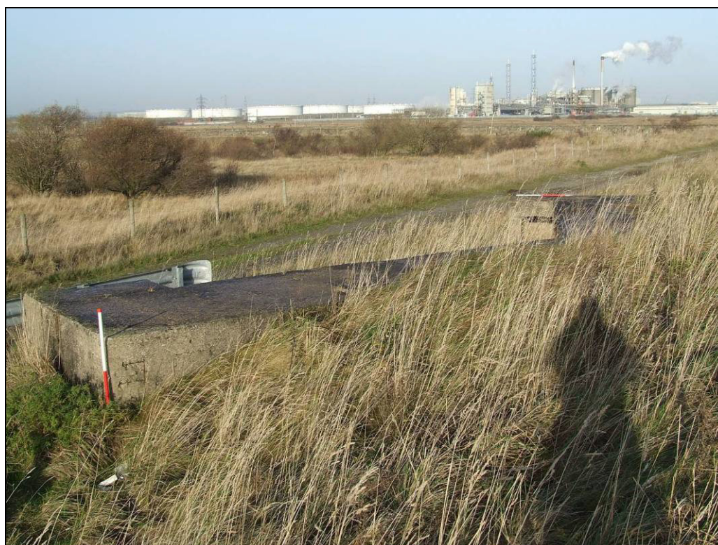
Fig 5.4.9 Partly buried section post (145) showing their distinctive chevron shape in plan.
