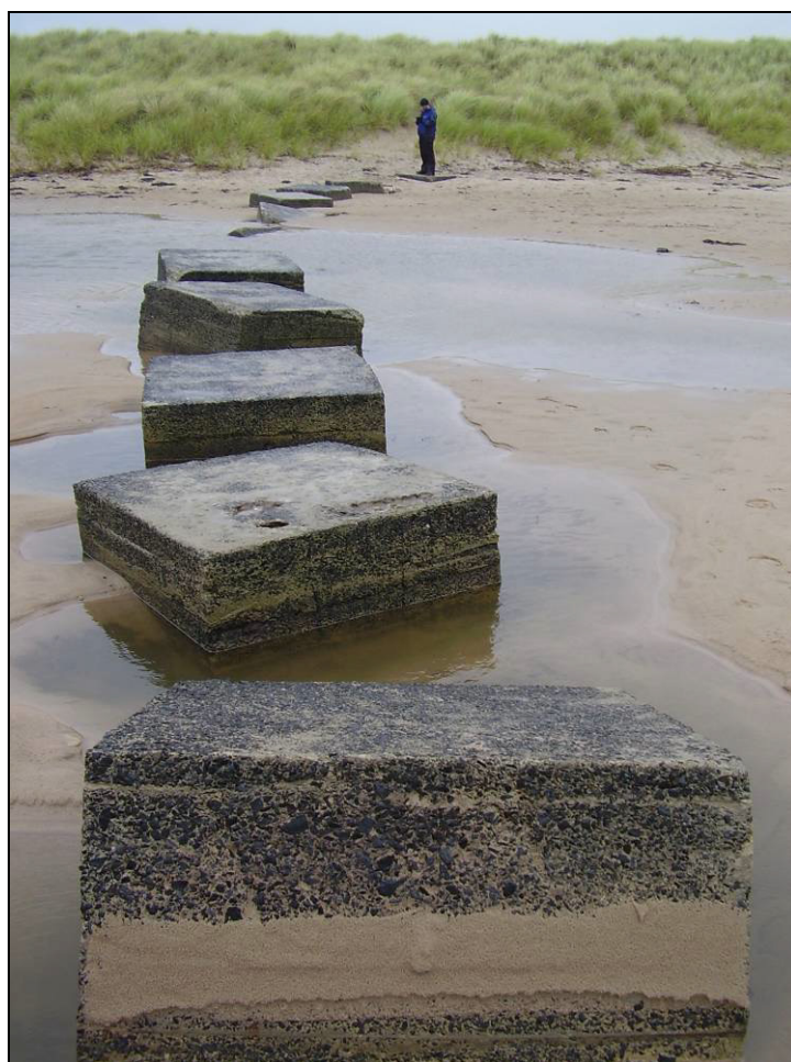
Fig 5.8.9 A line of 13 anti-tank blocks exposed in the mouth of a small burn.
