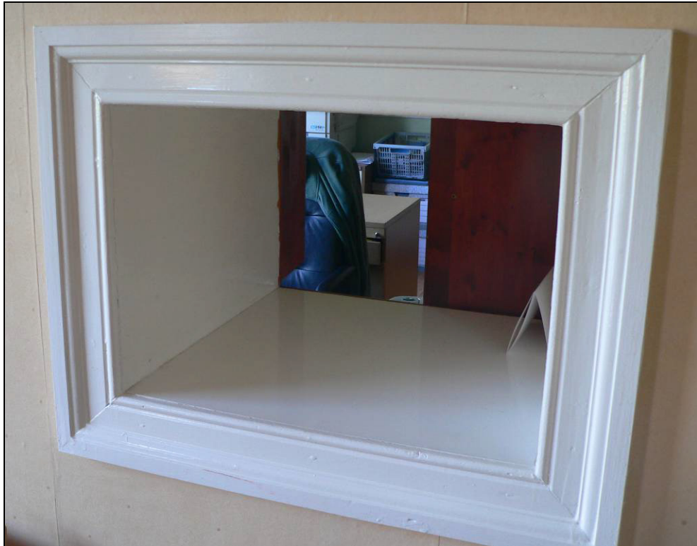
Fig 5.7.10 The serving hatch, showing the thickness of the interior walls.
