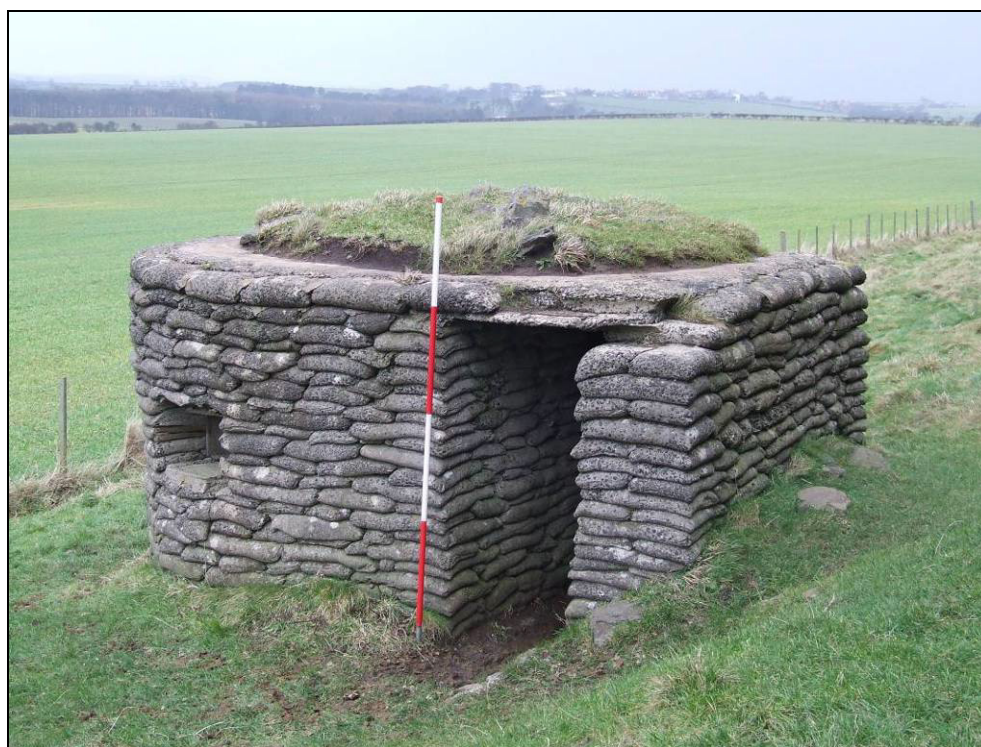
Fig.5.16.1 Pillbox constructed of concrete sandbags south of Dunstan Steads.
