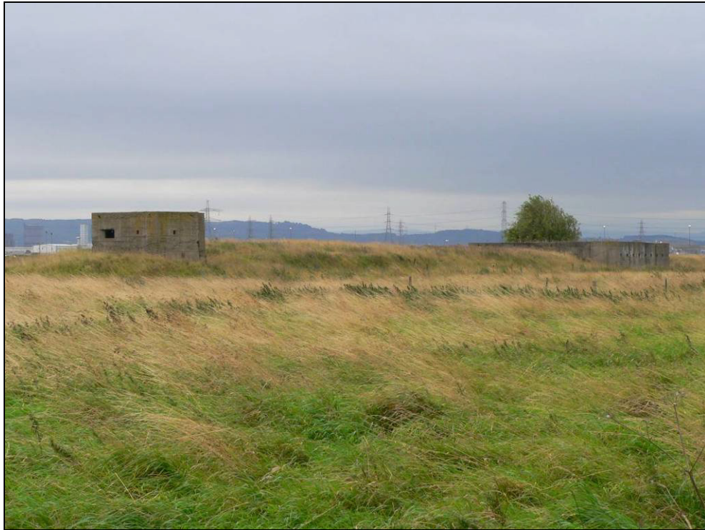
Fig 5.4.7 Former railway embankment reused as a platform for a pillbox (left) and section post (right).
