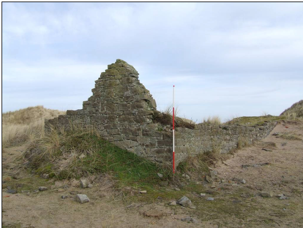
Fig 5.14.17 Partially upstanding gable end of Longhouse (409)
