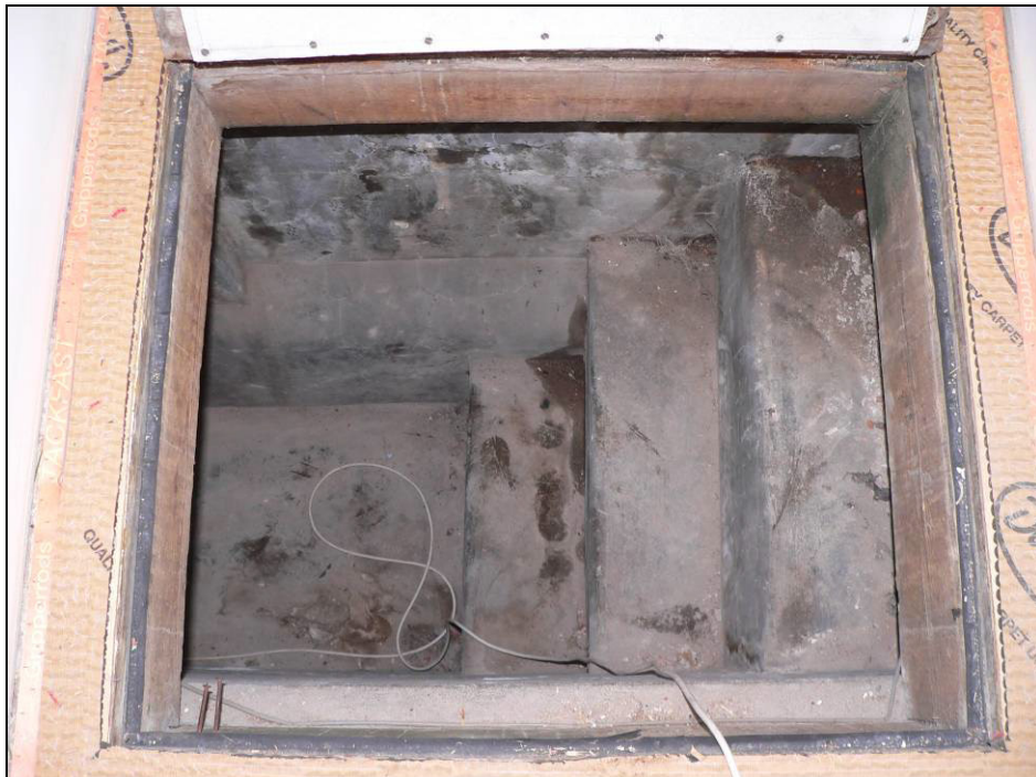
Fig 5.7.13 Hatch leading into basement level with concrete stairs.
