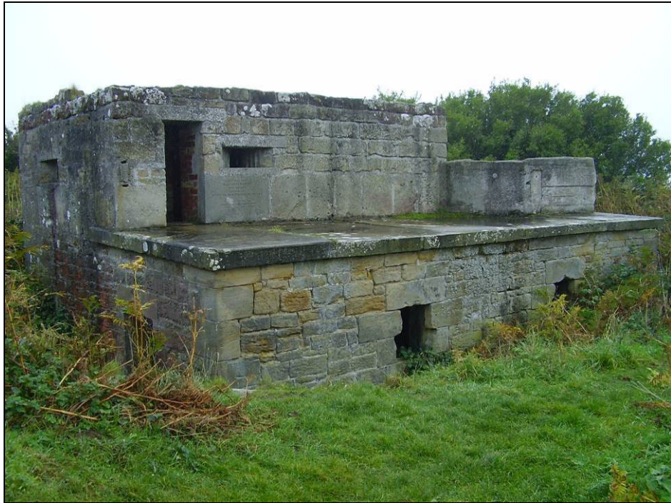
Fig 5.10.12 Alnmouth battery showing original features and later loop holes.
