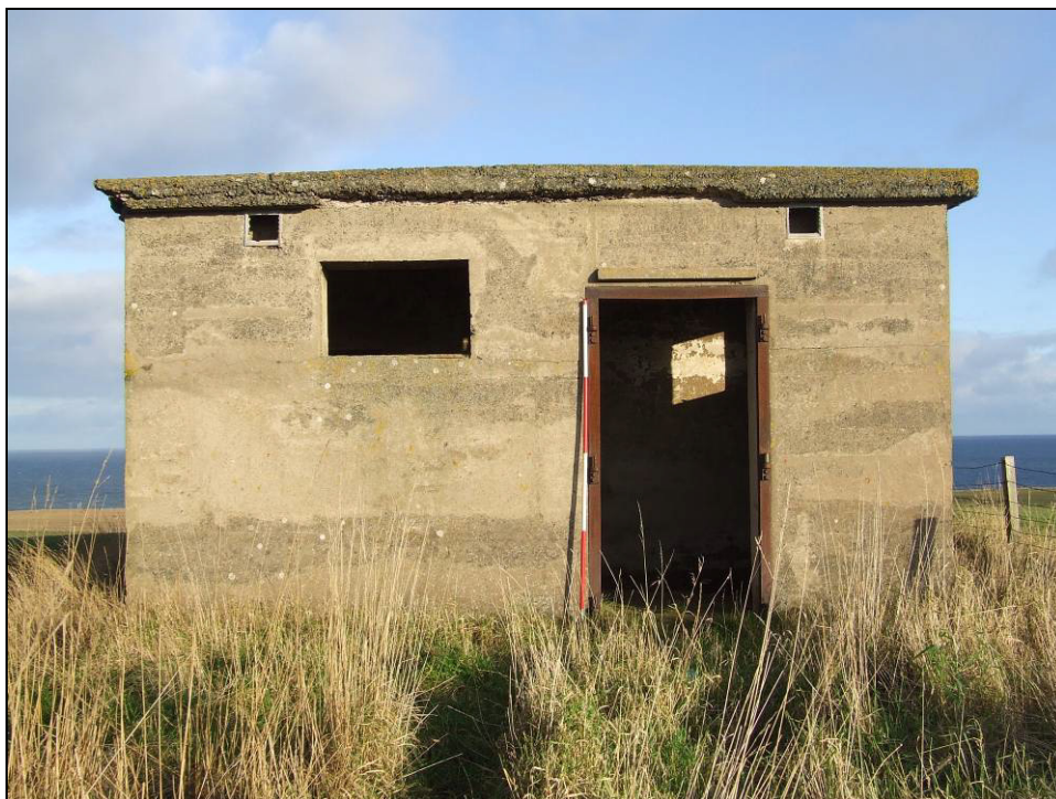
Fig 5.12.7 The Transmitter/Receiver block at the Scremerston radar station.
