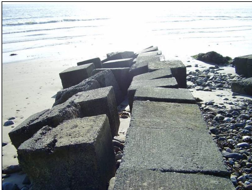
Fig 5.9.10 Anti-tank blocks used as part of the outflow of the Bondicarr Burn.
