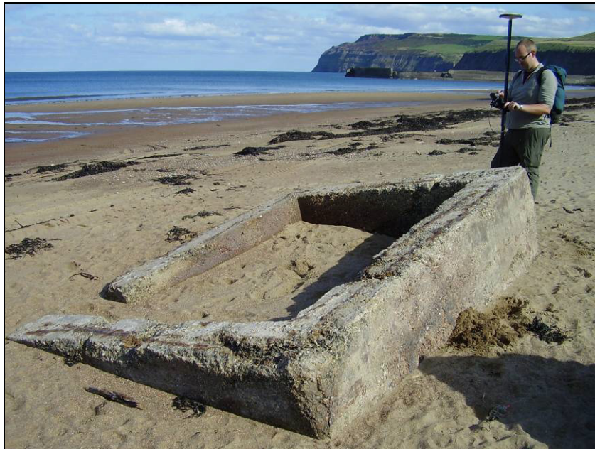
Figure 5.3.15 Slumped pillbox on the beach looking south towards Skinningrove harbour as seen in September 2009 .
