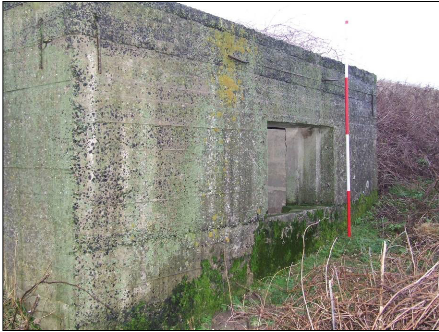
Fig 5.15.9 The front of the 6 inch gun emplacement (370)
