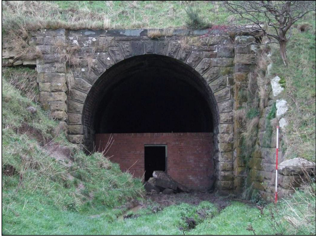
Figure 5.2.7 Tunnel mouth (422) at Kettleless end looking south.
