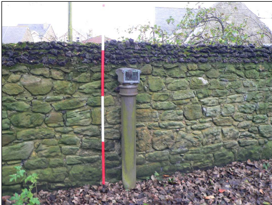
Fig 5.7.15 Possible ventilation pipe 437 against the inside of the south wall.
