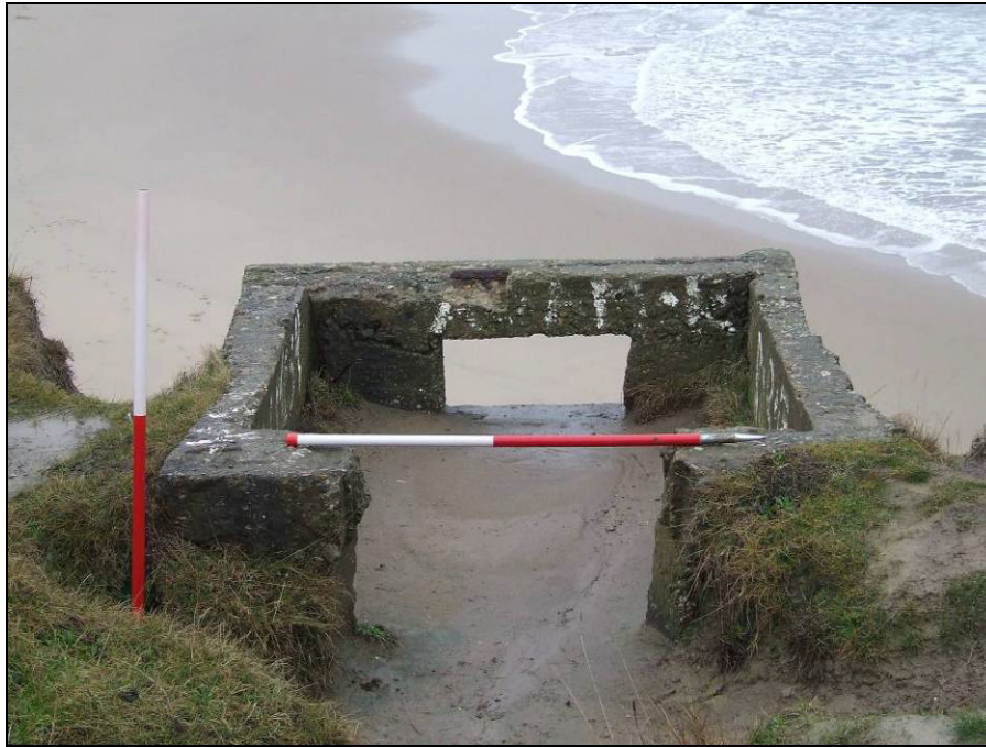
Fig 5.6.10 One of the eroding reinforced gun positions (129) overlooking the beach at Trow Point.
