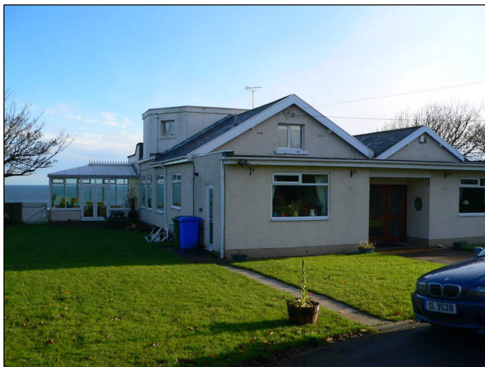
Fig 5.7.3 The former Officers Quarters and Observation Post at Robert's Battery.
