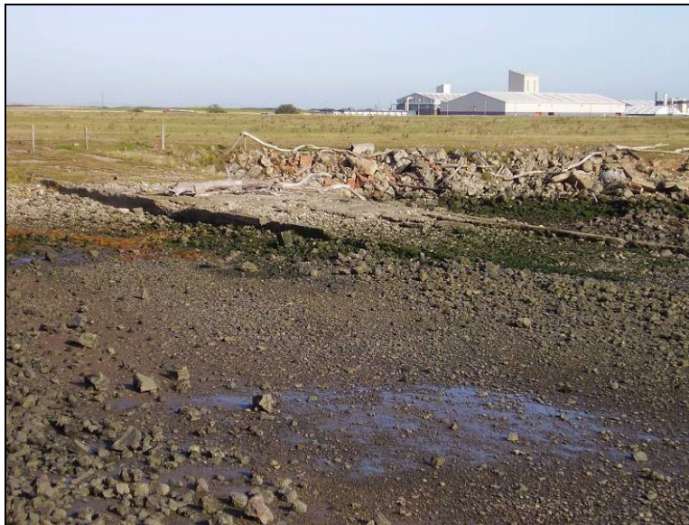
Fig. 7.19 The preserved slipway to the First World War seaplane base at Seaton Carew.
