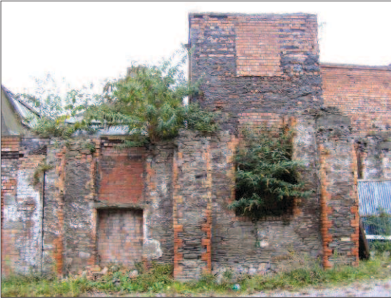
g) Area 3, standing building remains along the east face of Building 2, looking west.
