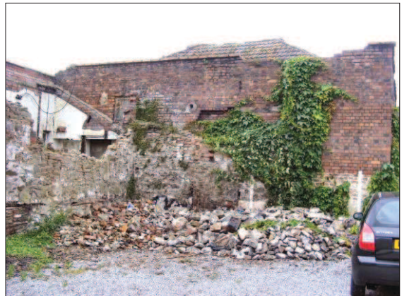
j) Buildings 6 and 7 from Area 6, looking west.
