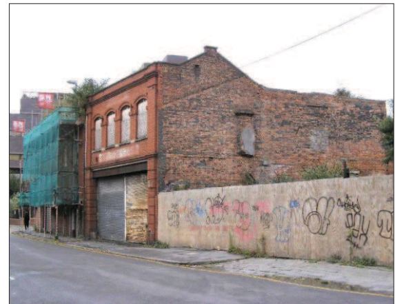
d) Building 2 and Area 3, Unity Street frontage, looking west.
