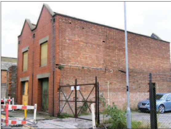
c) Building 2, Jacob Street frontage, looking south east.
