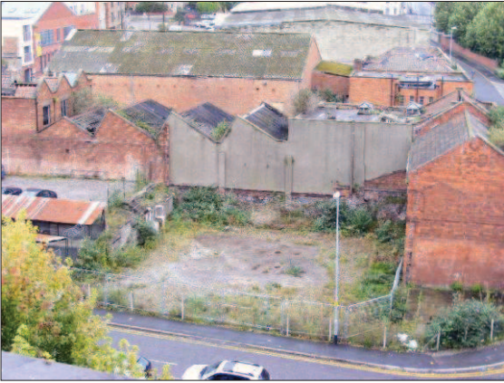
a) Aerial view part Hawkins Street frontage, with structures fronting Jacob Street/Unity Street. Looking east.
