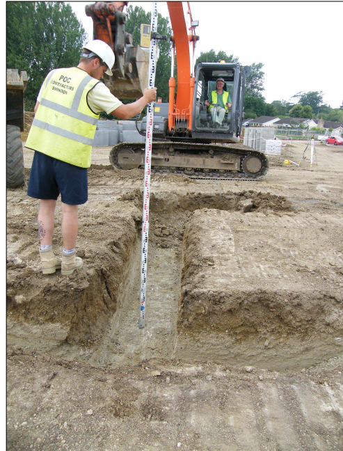
D) Detail of house foundations during excavation. Viewed from the east.
