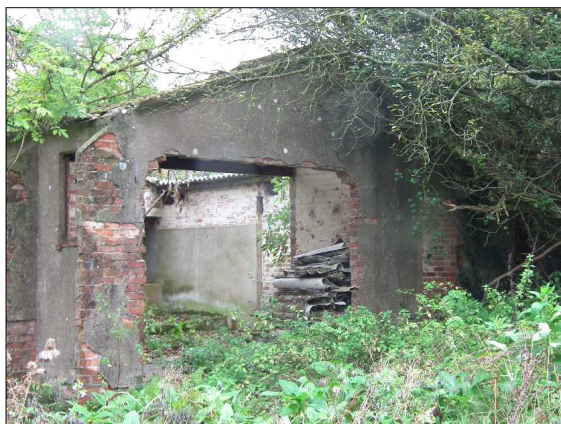
Plate c. The southern face of Structure 1, looking north-eastward.
