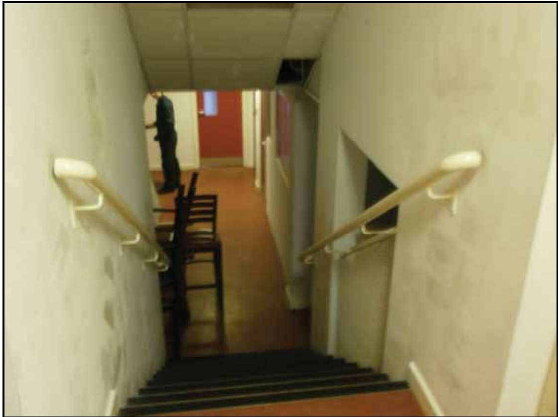
Pl. 17. The stairs down to the function hall from the lobby of the office building
