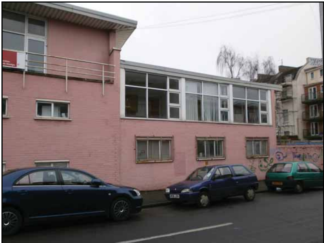
Pl. 16. The rear extension of the office building from Wilder Street
