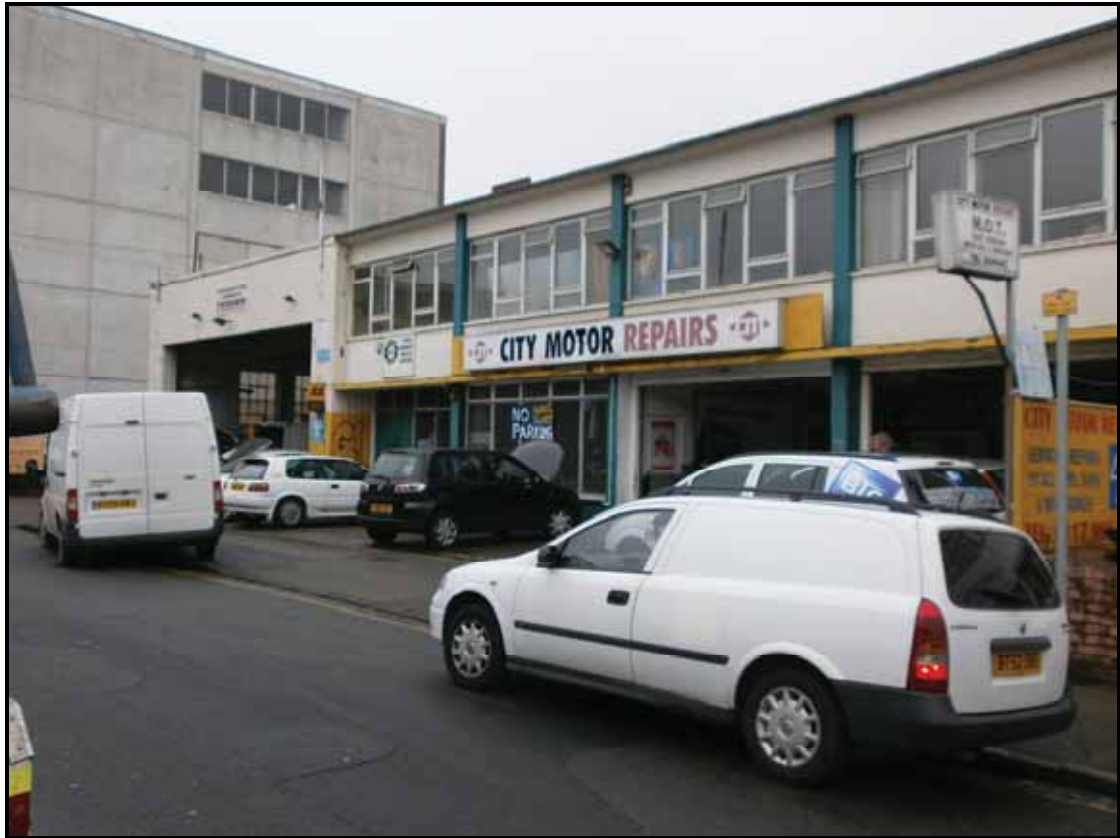
Pl. 3. The front of the garages from Dean Street
