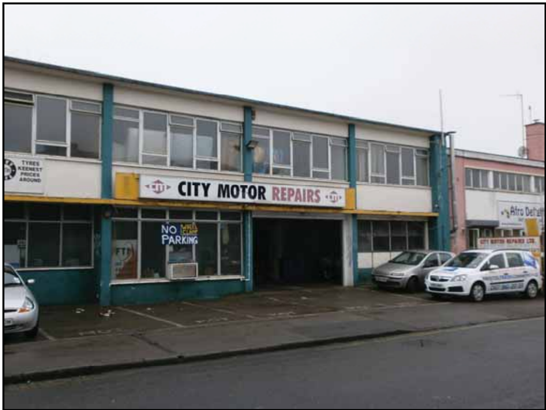
Pl. 10. The front of the garage building located in the middle of the block from Dean Street
