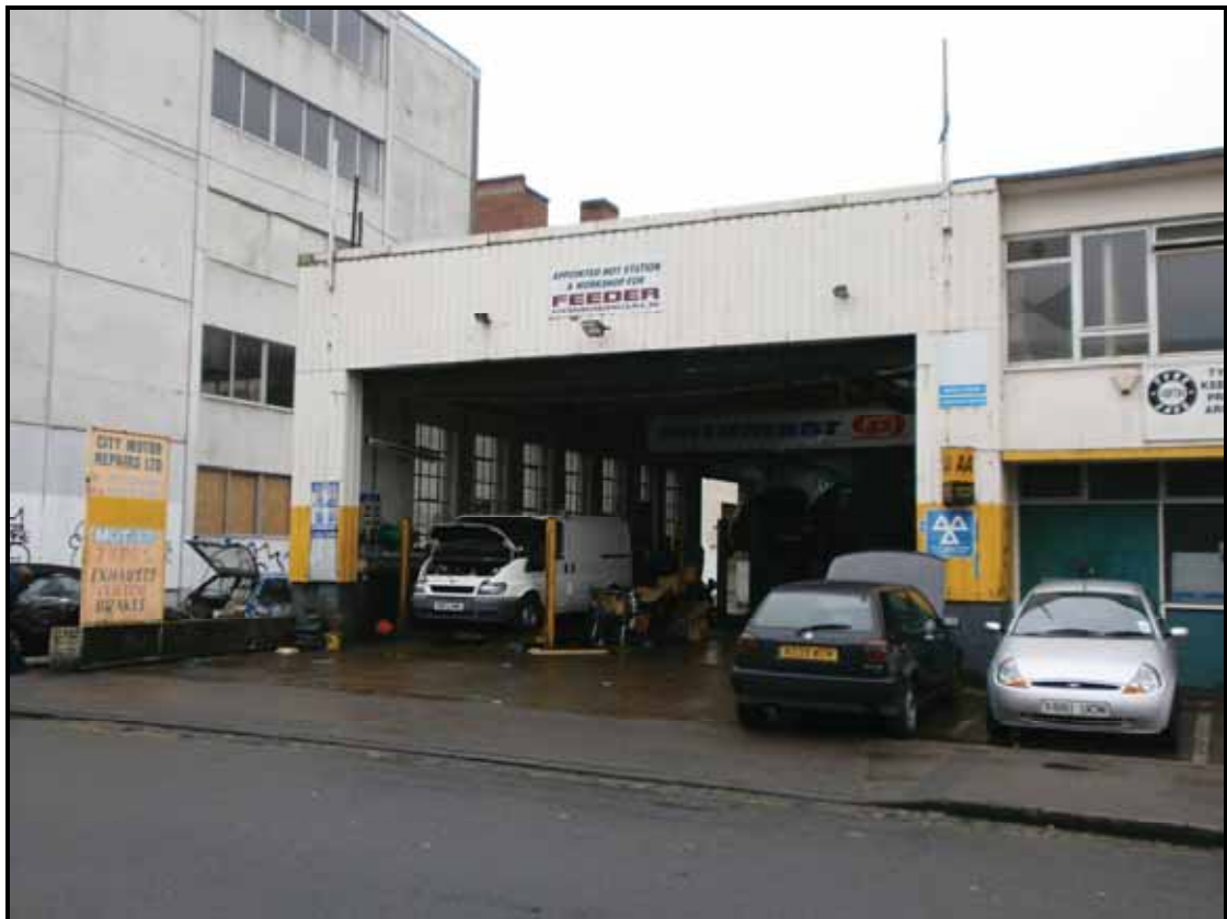
Pl. 6. The front of the garage on the corner of Chapter Street from Dean Street
