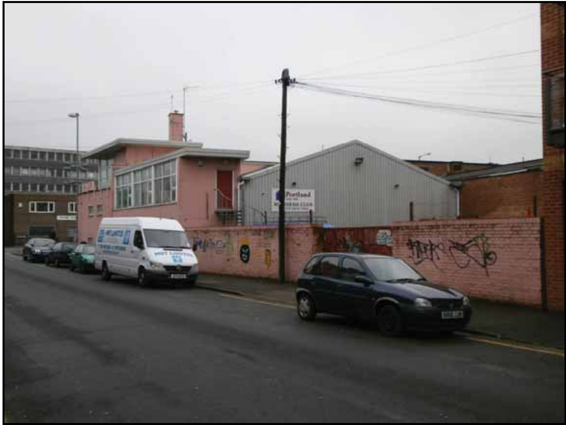
Pl. 5. View of the rear of the office building, extension and car park entrance from Wilder Street
