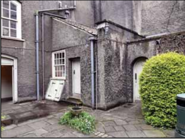
1. The small kitchen block attached to the NW corner of the chapel's northern wall, with cellar entrance beneath window. Note the stub wall marking its northern side, which may once have stretched the width of the northern courtyard, and marked the New Room's boundary with Pimm's Court beyond.
