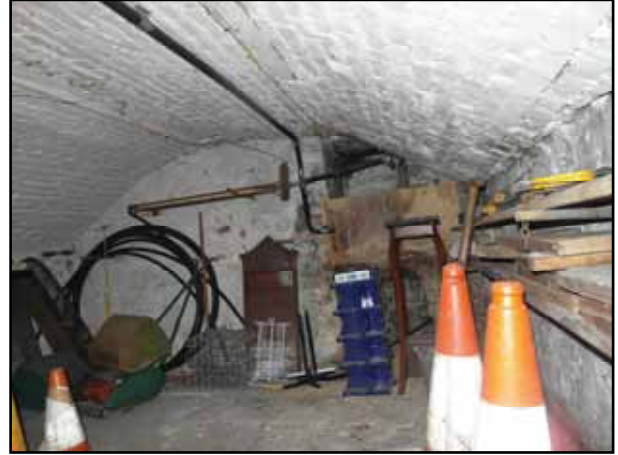
2. Vaulted brick cellar underneath the kitchen block. View to NNW.
