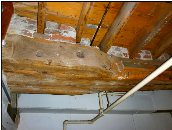
3. One of the many massive timbers, this one tied with iron bolts or nails, acting as floor joists within the surviving historic parts of the warehouse, units 3 and 4. The appearance of some of these features suggests that they may be reused ship's timbers.
