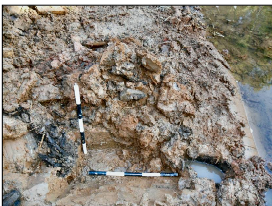
f) West end of Wall 519, from west, showing stepped foundation course and adjacent post-holes, Contexts 516 and 517. Scales: 500mm.
