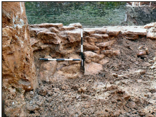
d) Detail of butt joint between Wall 518, to left and Wall 519, to right, facing south. Scales: 500mm.
