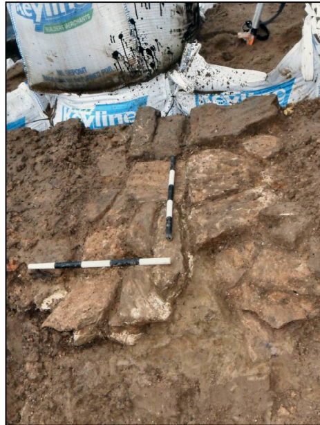
j) Butt joint between Wall 601, in Cut 607, to right and Wall 602, in Cut 605, to left. Viewed from south. Scales: 500mm.
