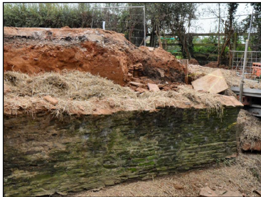
c) North-east facing view of section through redeposited clay to rear (north) of north abutment (Context 129), showing location of Masonry 528. No scale.
