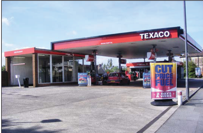
a) General view of study site from south, showing location of access to underground storage tanks to left of frame, house on Broncksea Road in background.
