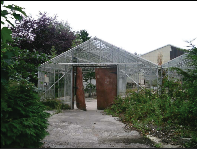
a) Westernmost greenhouse, with encroaching vegetation, looking north-east.
