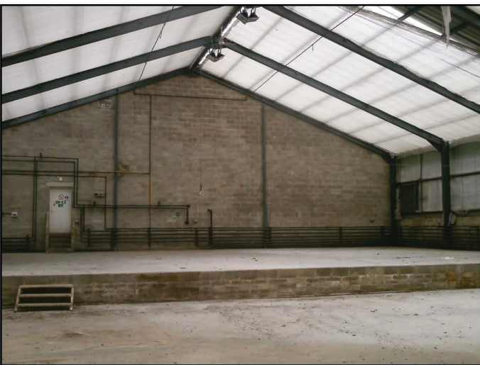
c) Internal view of warehouse, looking north, showing that rear portion of building is raised, due to sloping nature of site. The offices referred to in the text are located beyond the wall in the background.
