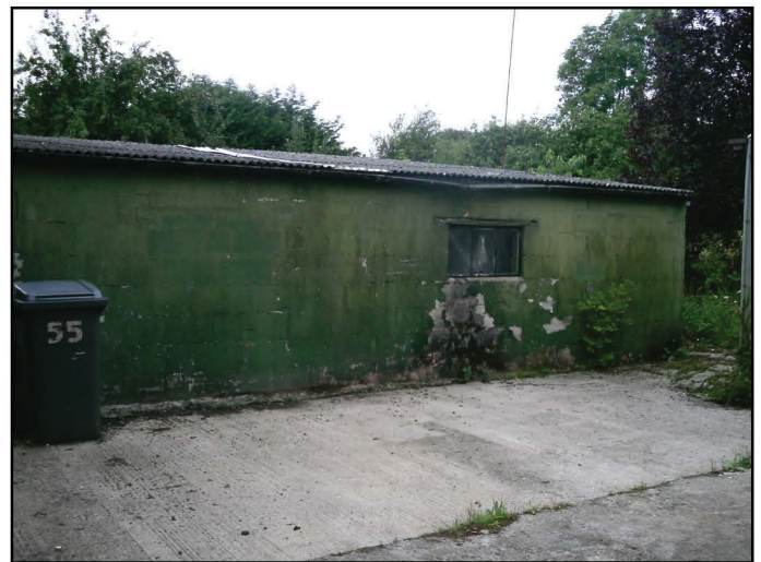
d) Concrete block shed, at south-western corner of greenhouses, from west.
