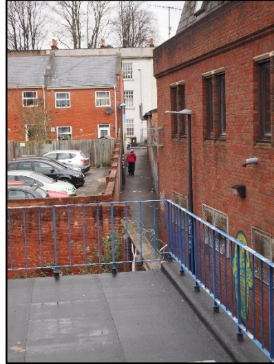
8) View of the public footpath where it emerges from between Nos. 81 and 83 and continues towards Wilson Street, looking northwest
