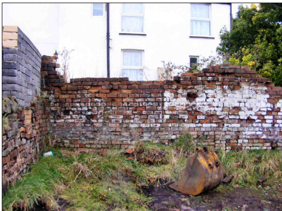
e. Building scars, and paint on the southeastern boundary of the Study Area, looking east.
