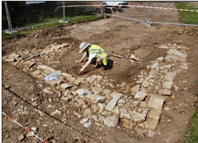
Plate 2. Structure 'A' looking northeast
