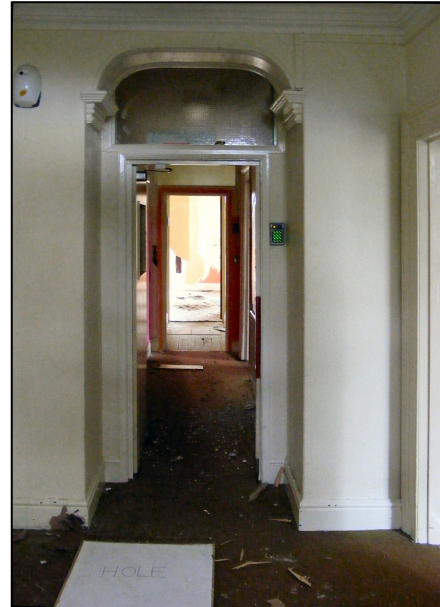
Plate 16. Looking south at internal doorway from the entrance of Concorde Lodge
