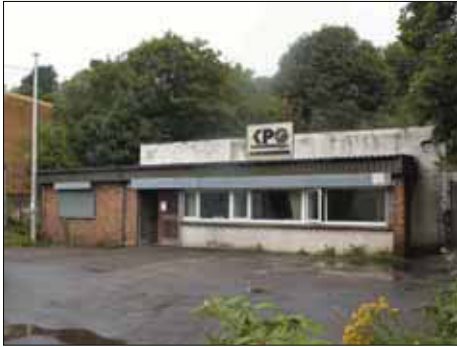
Plate 1: Crews Hole Road frontage of the modern breezeblock and brick engineering works, viewed from the south
