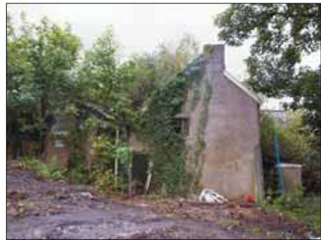
Plate 6: rear view of the derelict former inn, viewed from the north
