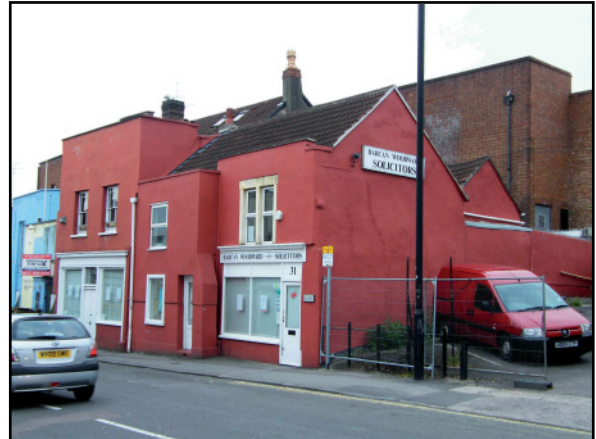
2. Offices of Messrs Barcan Woodward, Solicitors, North Street, Bedminster. View to south-east.
