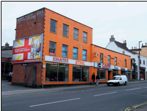
3. Premises of Carr Power Products, North Street, Bedminster. View to south-west.
