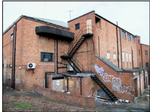
4. South-eastern, rear elevations of Gala Bingo Hall. View to north-west.
