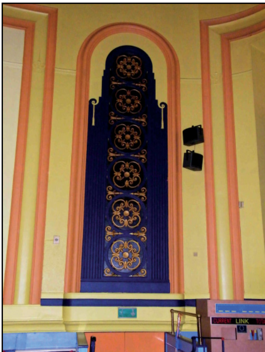
14. Gala Bingo Hall, detail of decorative air extraction grille, main auditorium, lower (stalls) level.
