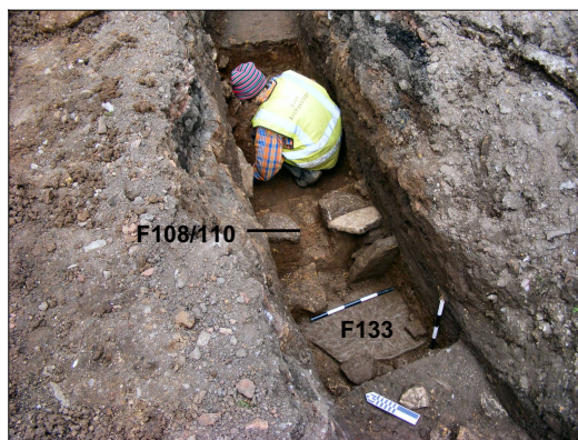
Plate 5. Trench D stone lined base and remnants of edge-on stones defining northern side of culvert F133 truncating southern side of bank makeup F108/110, viewed from the west, scale 500mm x 500mm
