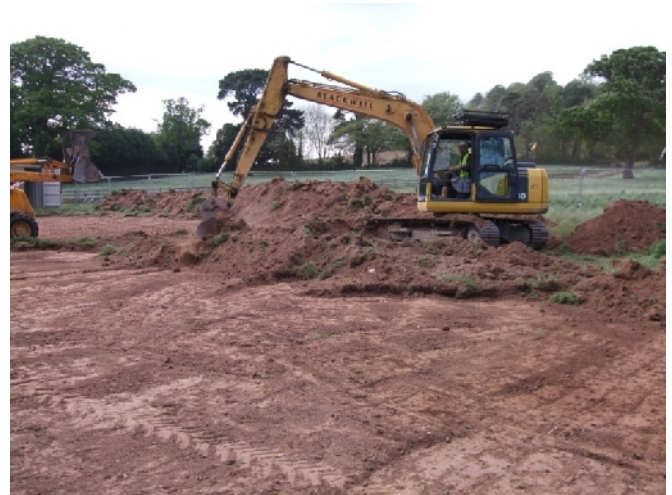
Plate 4. General site conditions stripping site compound (southern end of scheme)
