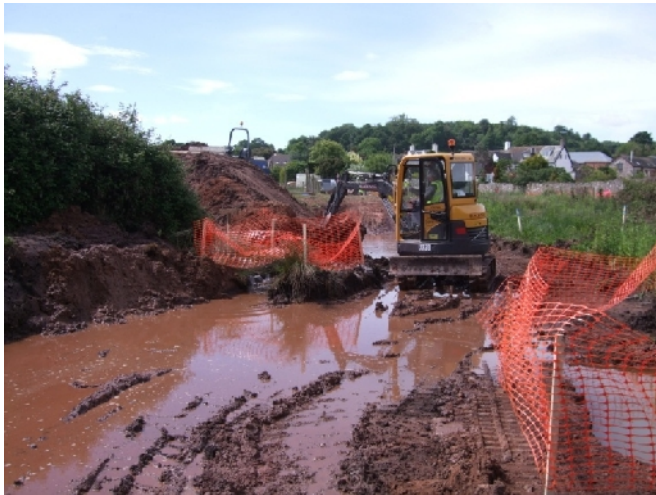
Plate 3: General site conditions (northern end of scheme)
