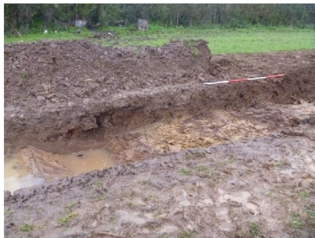
Plate 3. [1003] excavated, [1005] exposed (from W; 2m scale)
