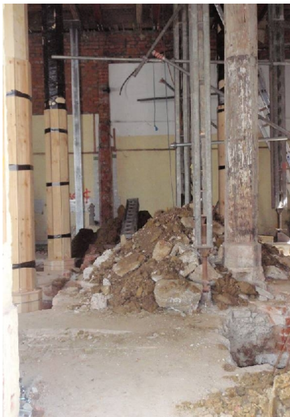
Plate 2. Interior showing replacement pillars and surviving original pillar (right; from S)
