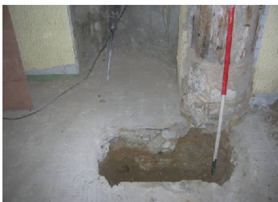
Plate 7. Trench 5, general (from N)
