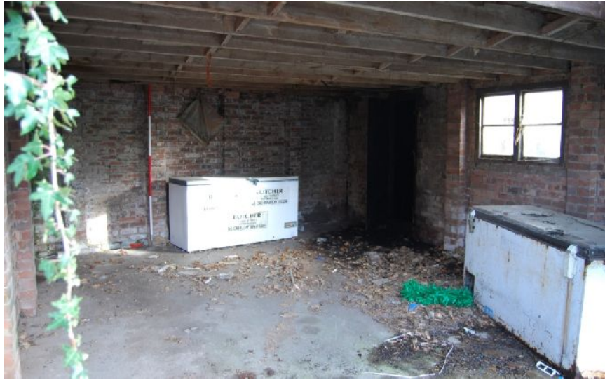
Plate 25. Building 4, ground floor (from SW; 2m scale)
