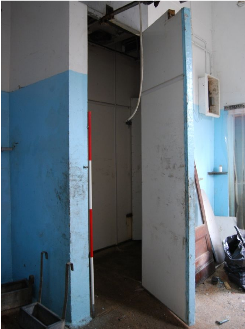
Plate 9. Building 1, south room (from N; 2m scale)
