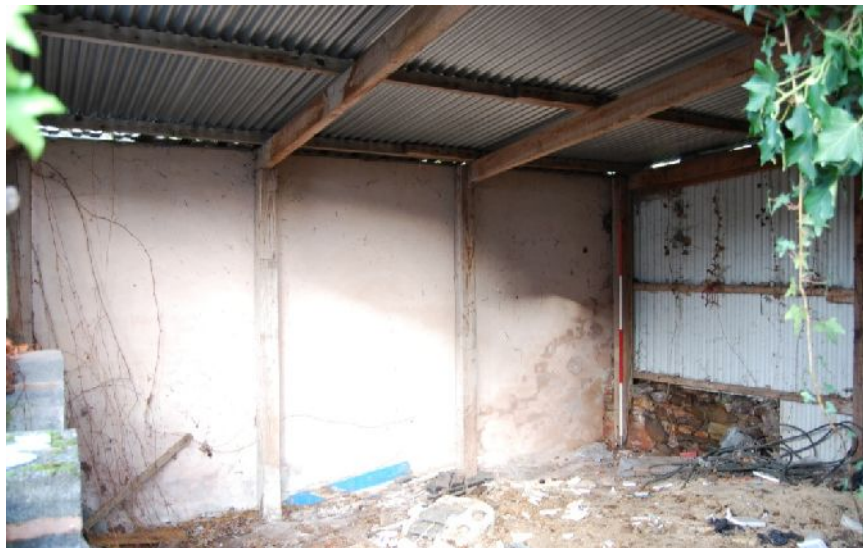
Plate 27. Building 4, lean-to (from S; 2m scale)
