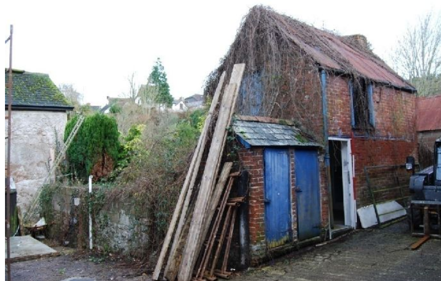
Plate 16. Building 2 (from S; 2m scale)
