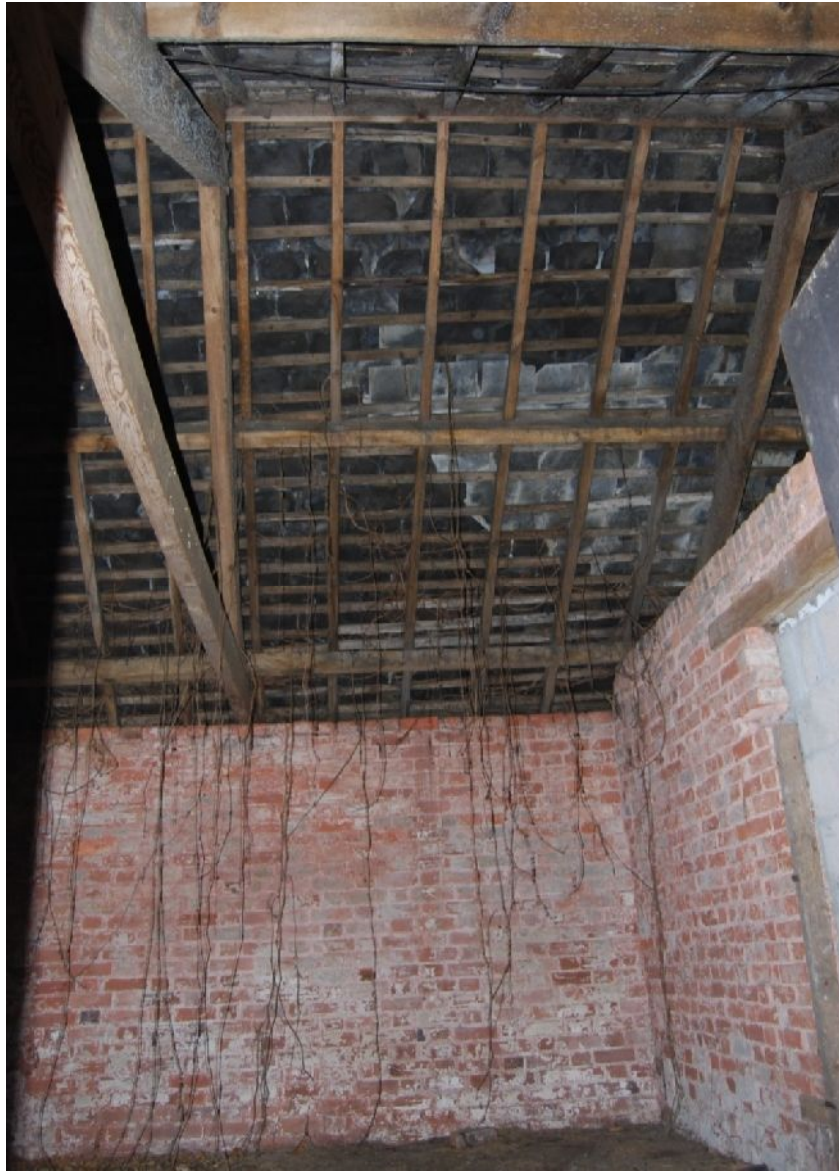
Plate 13. Building 1, 1 st floor (from NW; no scale)
