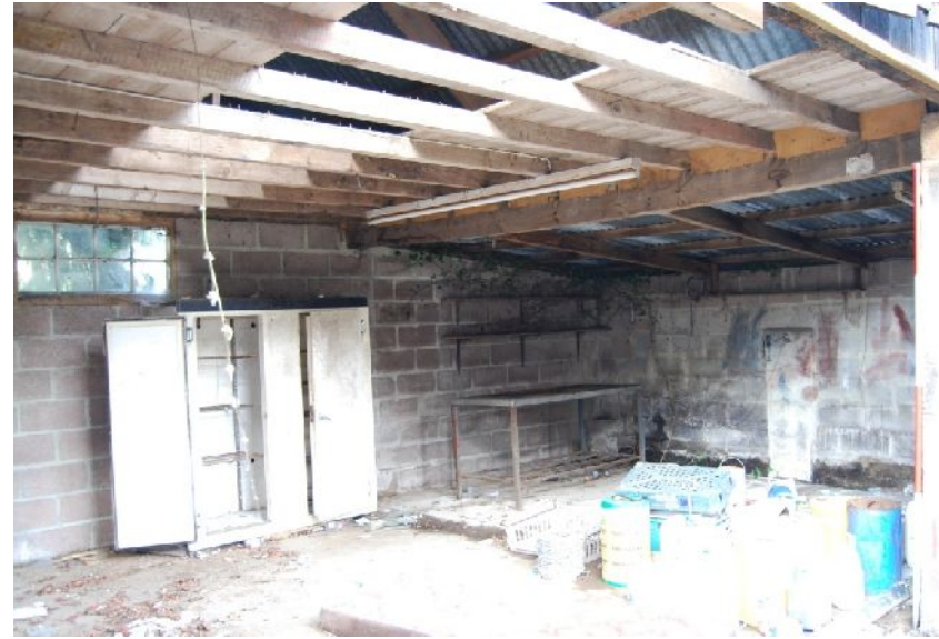
Plate 22. Building 3, interior (from S; 2m scale)
