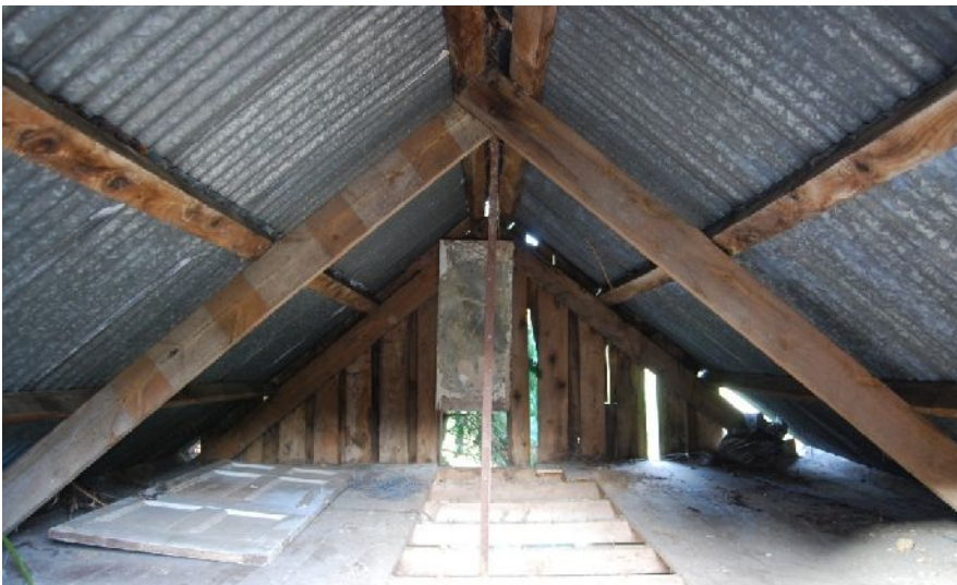
Plate 23. Building 3, roof space (from SE; no scale)
