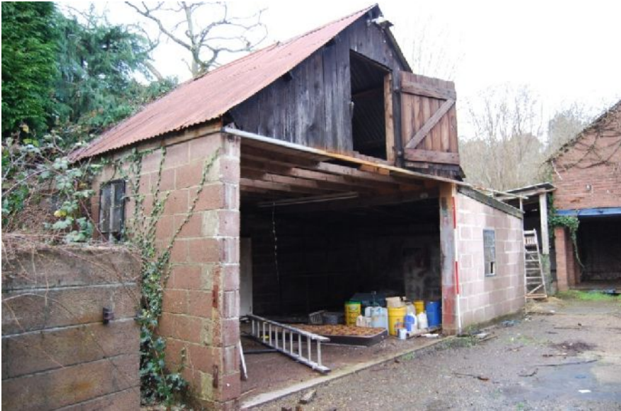
Plate 21. Building 3 (from S; 2m scale)
