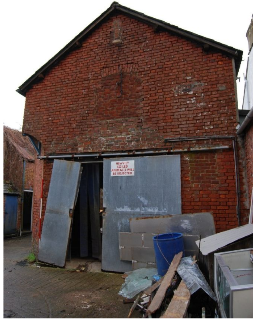
Plate 2. Building 1 gable (from SSW; 2m scale)
