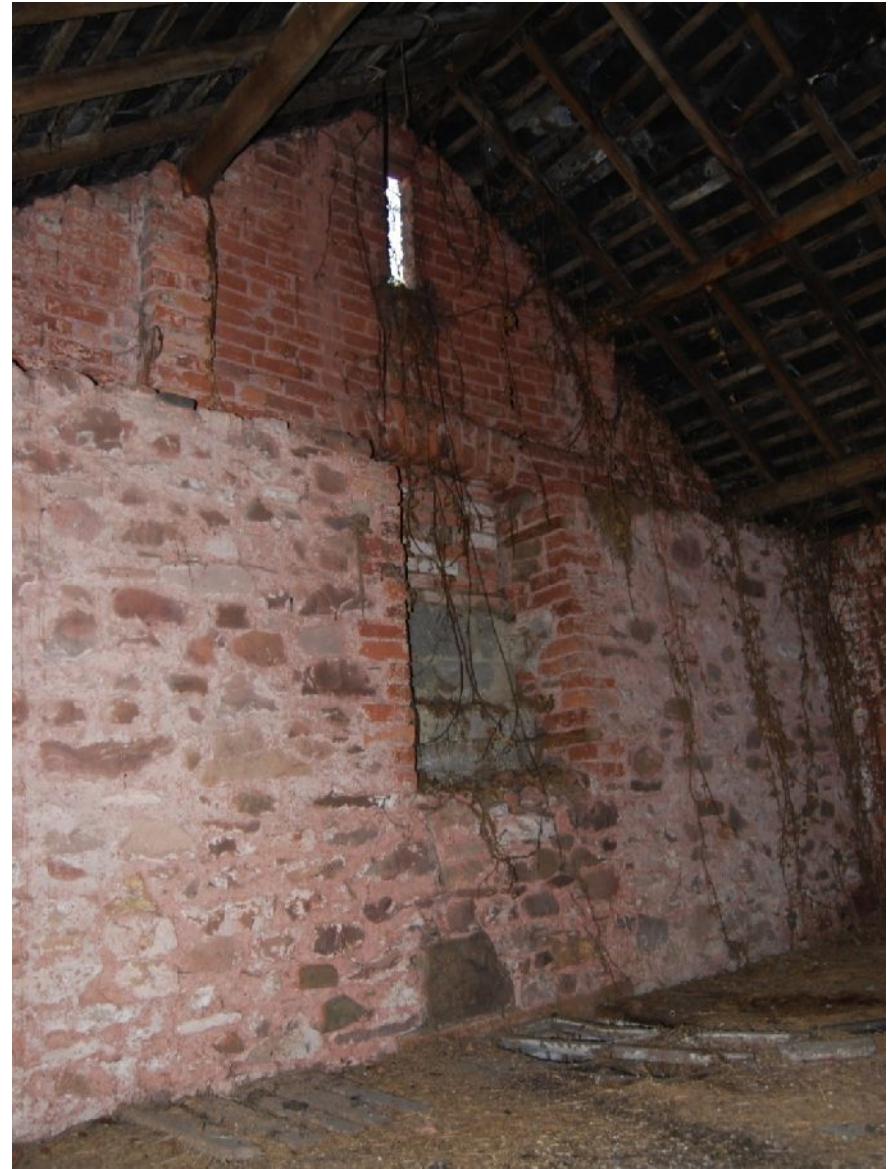
Plate 12. Building 1, 1 st floor (from WSW; no scale)
