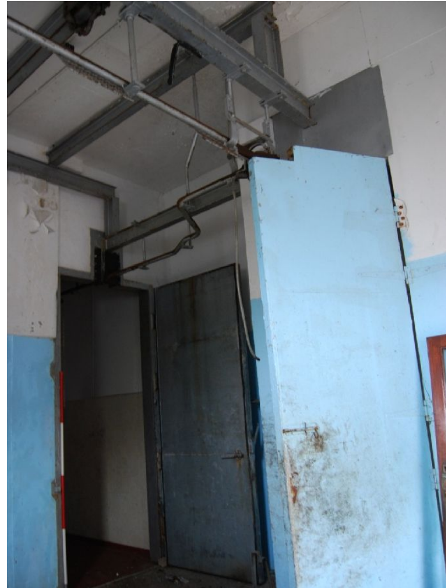
Plate 8. Building 1, south room showing rail and frame (from W; 2m scale)
