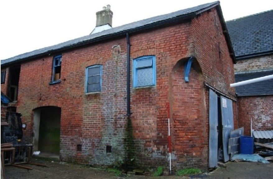
Plate 3. Building 1 exterior (from WSW; 2m scale)
