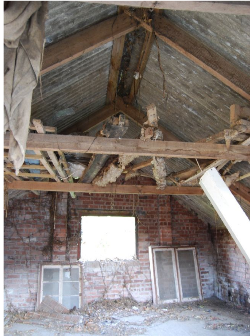
Plate 26. Building 4, 1 st floor (from SSW; 2m scale)
