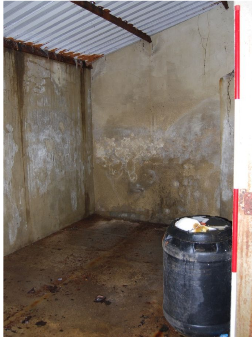
Plate 14. Building 1, lean-to (from NNE; 2m scale)
