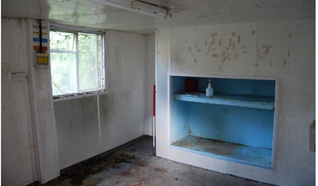
Plate 18. Building 2, ground floor (from S; 1m scale)
