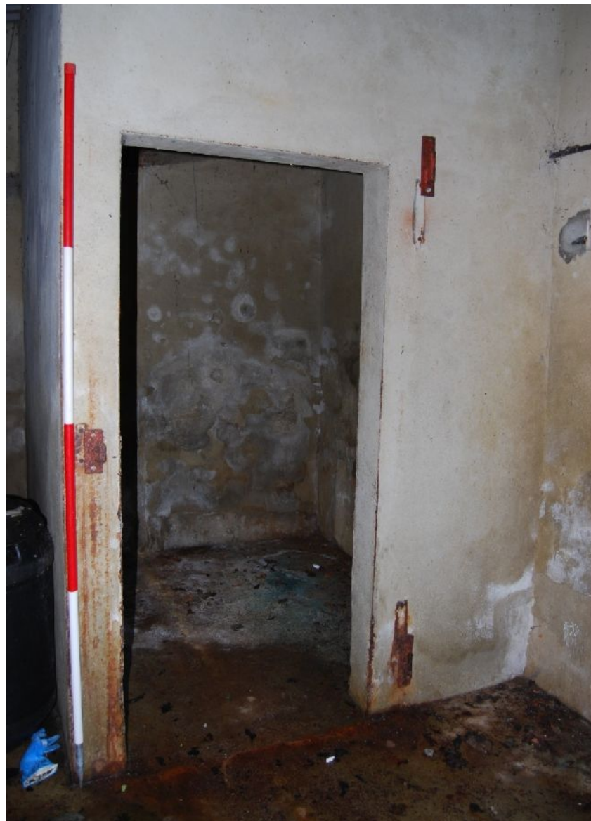
Plate 15. Building 1, lean-to cubicle (from NNW; 2m scale)
