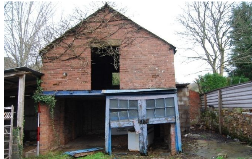
Plate 24. Building 4, roof space (from SSW; 2m scale)
