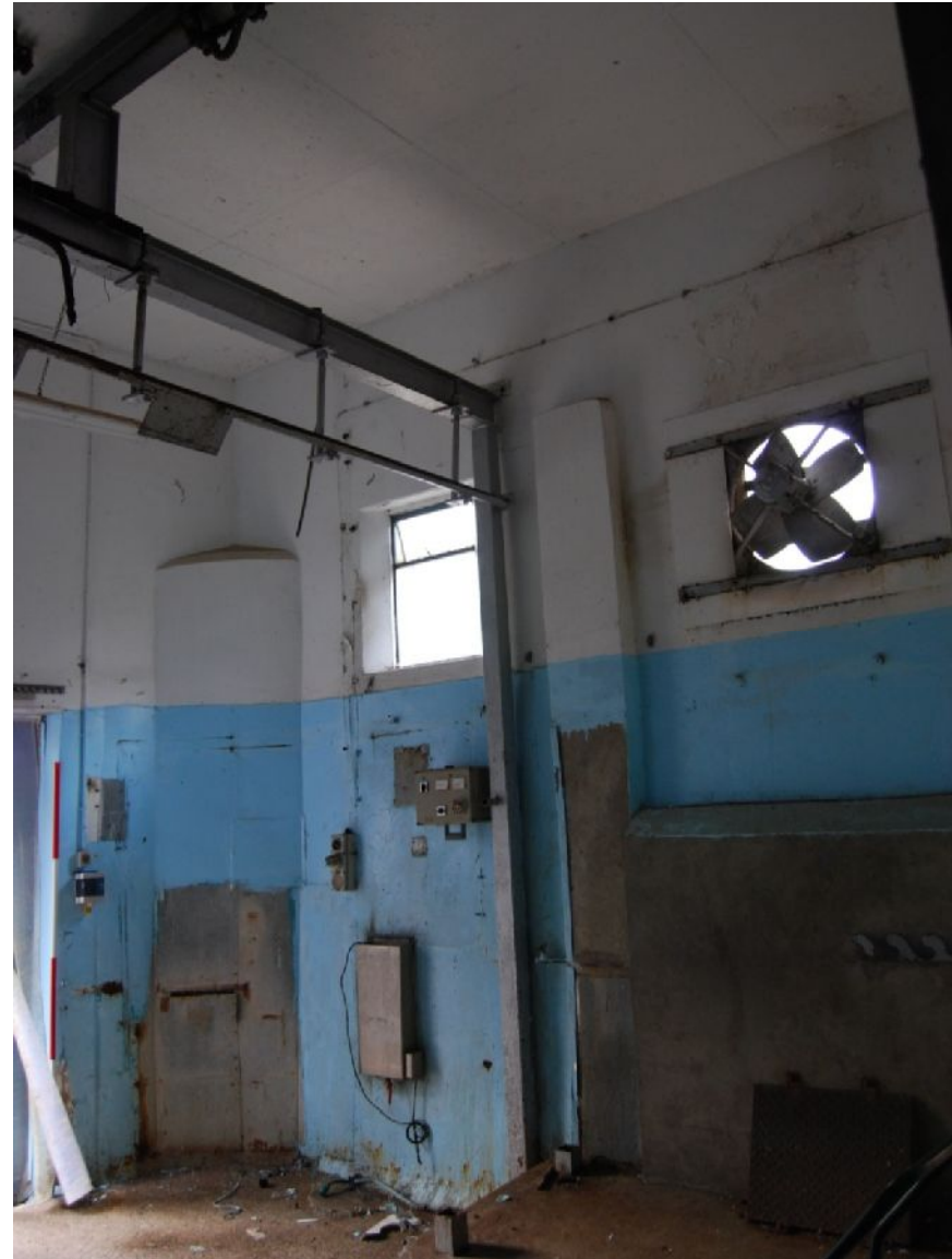
Plate 10. Building 1, south room showing rail and frame (from E; 2m scale)
