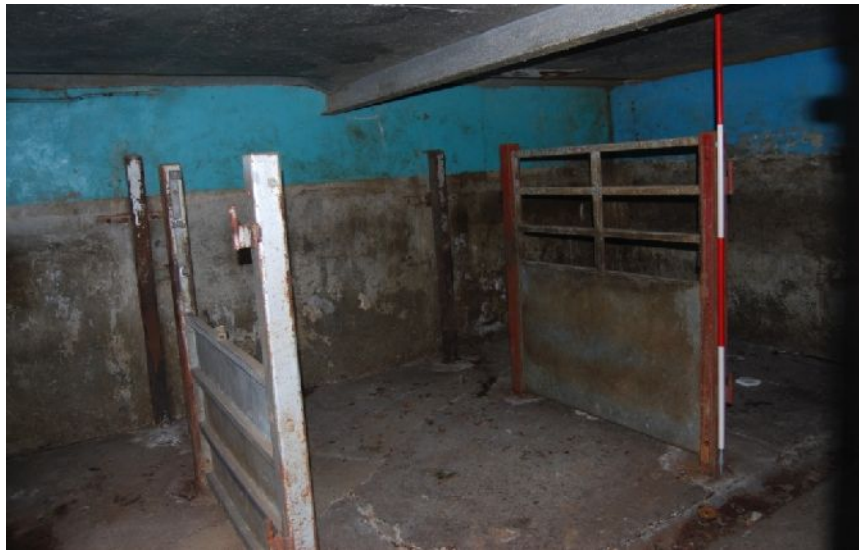
Plate 6. Building 1, north room (from W; 2m scale)
