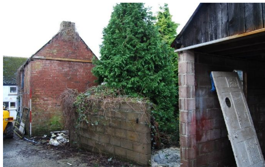
Plate 17. Building 2 in relation to Building 3 (from NE; 2m scale)
