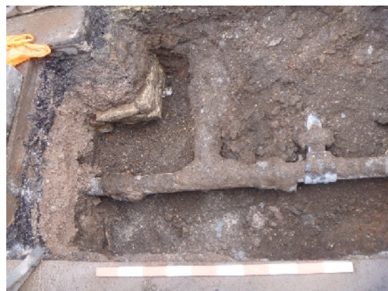
Plate 6. Pit 31 showing foundation (3106) (from N)
