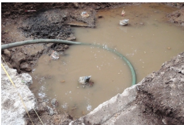
Plate 6. Timbers in situ (protected by plastic bags)
