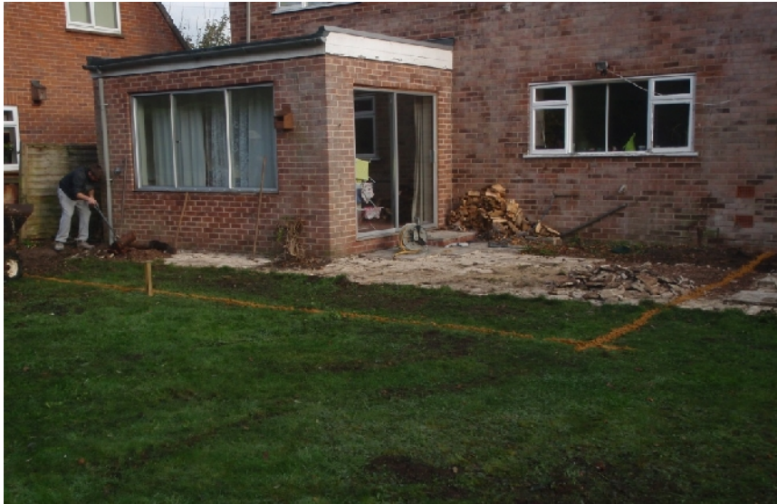
Plate 1. General location of foundation trench (from SE)
