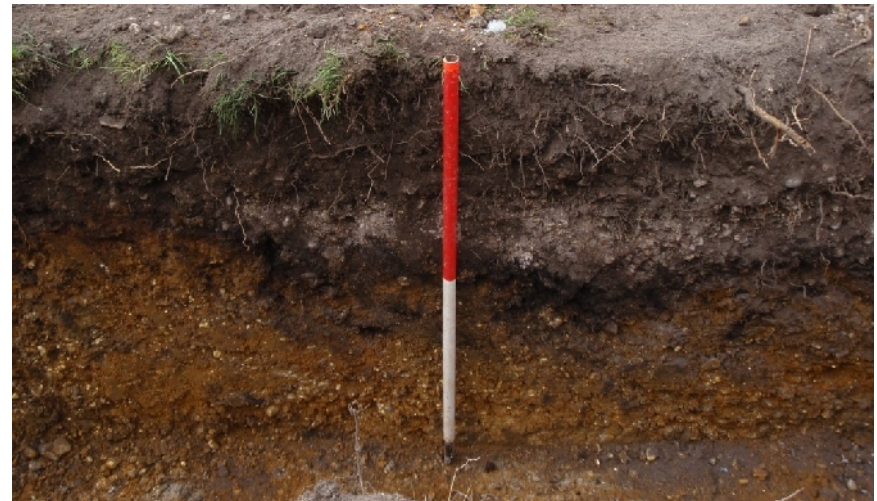
Plate 4. Foundation trench profile (from N)
