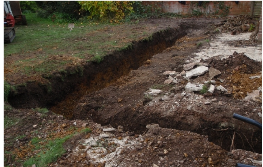
Plate 2. Excavated foundation trench (from SW)
