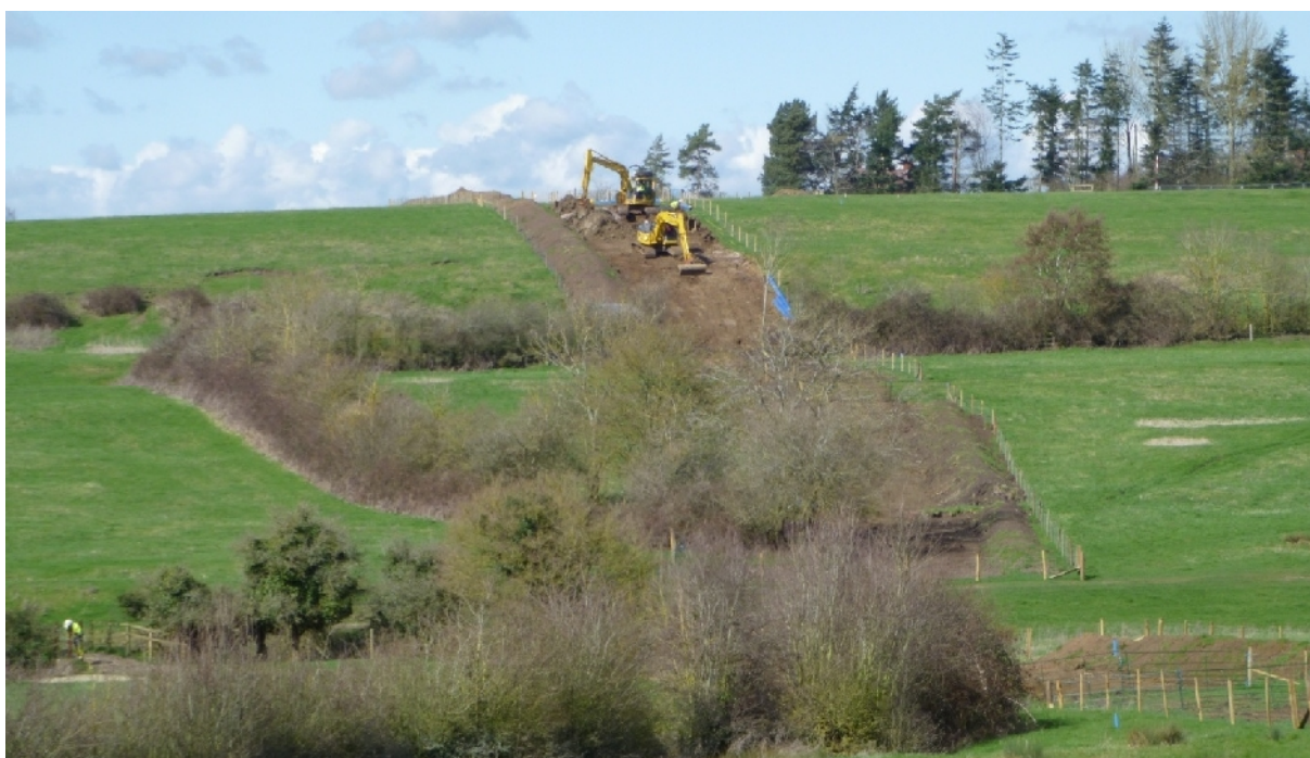
Plate 2. Work in progress on Chilvester Hill (from SE)
