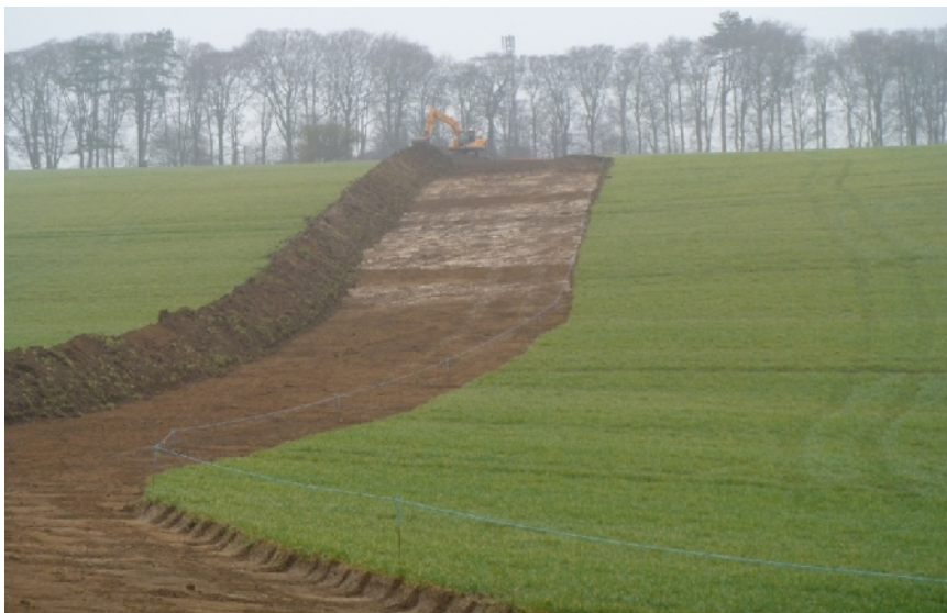
Plate 3. Easement at Bulbridge (from SE)
