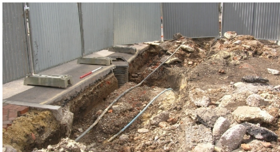
Plate 3. Service trench (from NE)
