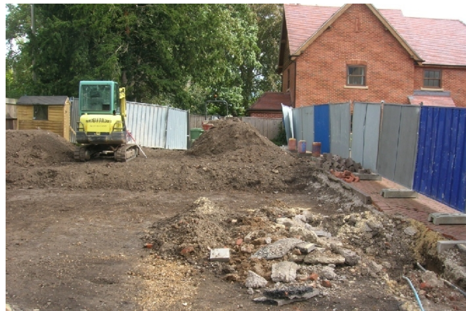
Plate 2. Service trench and beyond (from W)
