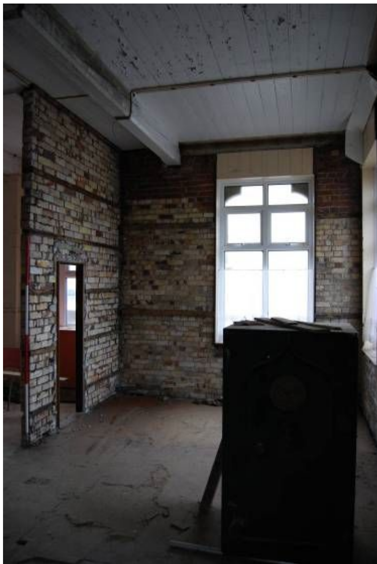
Plate 11. Area 1, office and safe (from SSE; 2m scale)
