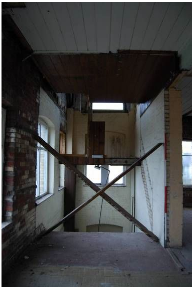
Plate 27. First floor, stairwell (from NNW; 2m scale)
