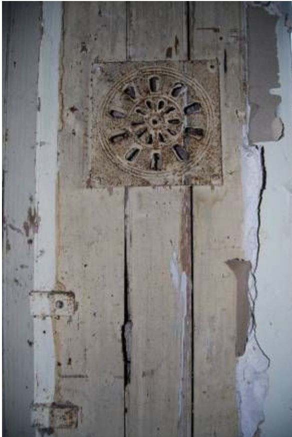
Plate 37. Air vent, Area 7 (from SSE; Figure 4 )
