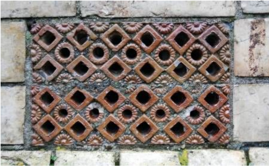
Plate 6. The Site exterior, ceramic vent (from NNW; no scale)
