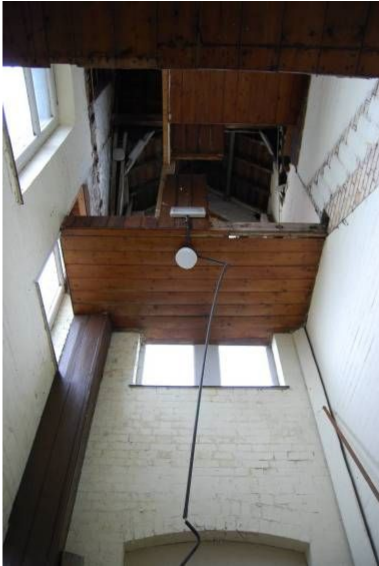
Plate 13. Area 2, stairwell, looking up (from NNW; no scale)
