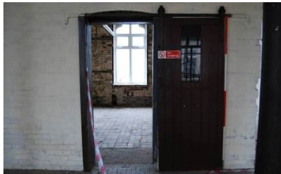
Plate 16. Area 4, access via sliding door (from NNW; 2m scale)
