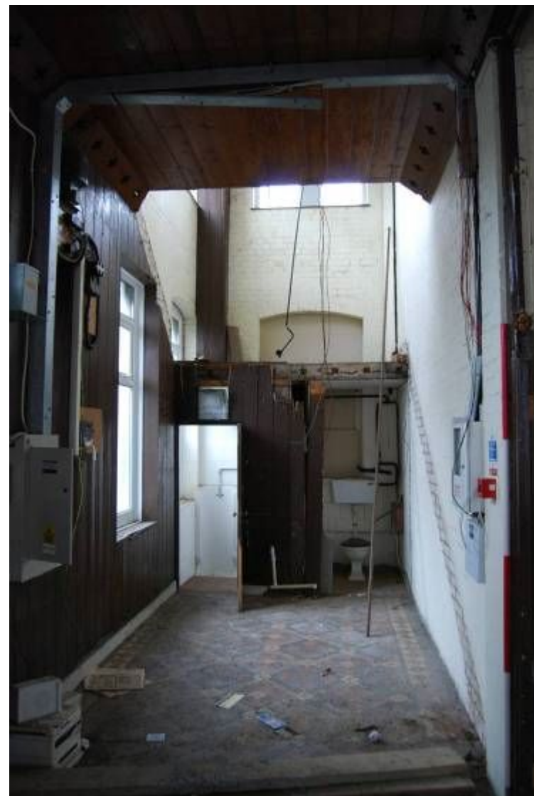
Plate 12. Area 2, stairwell (from NNW; 2m scale)
