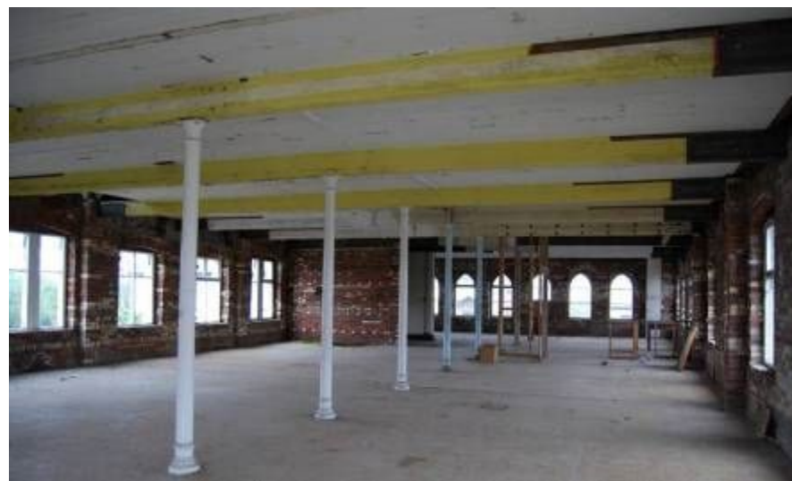
Plate 26. First floor (from NE; 2m scale)
