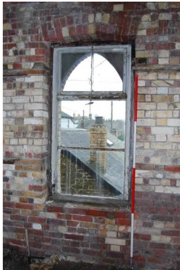
Plate 28. First floor, west gable window (from WNW; 2m scale)
