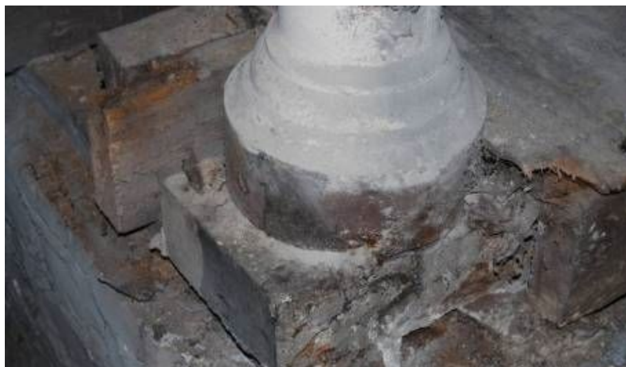
Plate 20. Area 7, column base (from SW; 2m scale)
