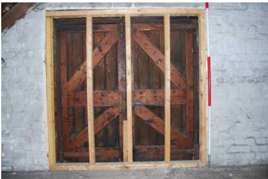
Plate 35. Second floor, east gable goods access (from WSW; 2m scale)
