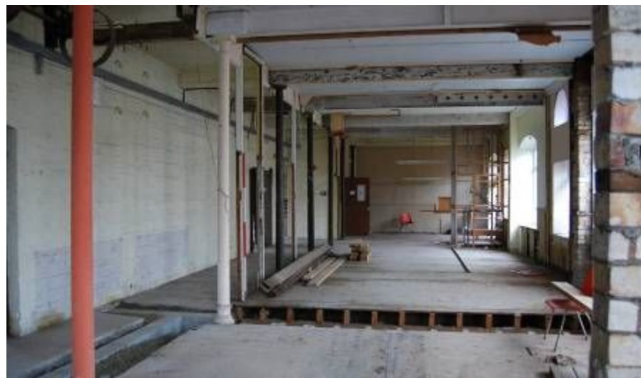
Plate 19. Area 7 showing cast iron columns (from ENE; 2m scale)
