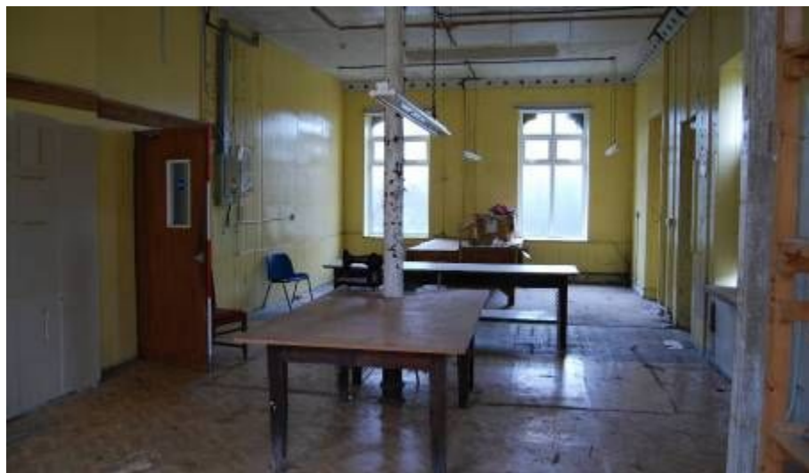
Plate 18. Area 6 (from NNW; 2m scale)
