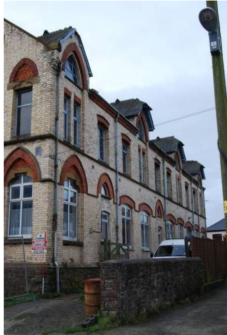
Plate 5. The Site exterior (from NE; 2m scale)
