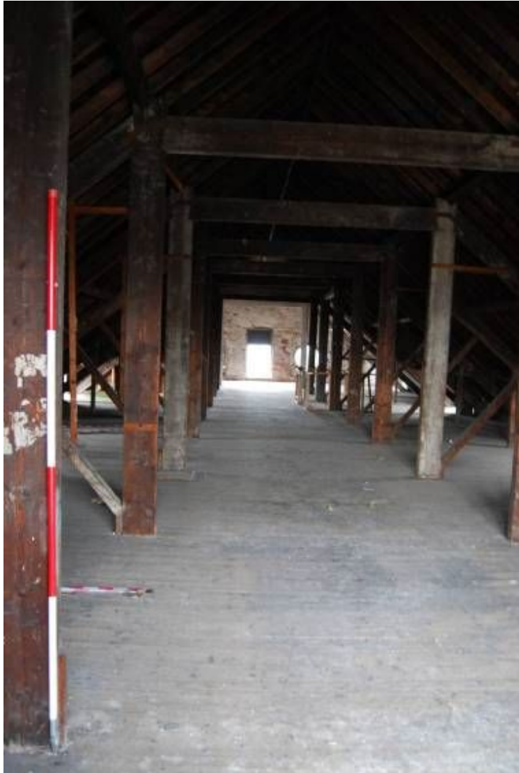
Plate 31. Second floor, bays (from ENE; 2m scale)
