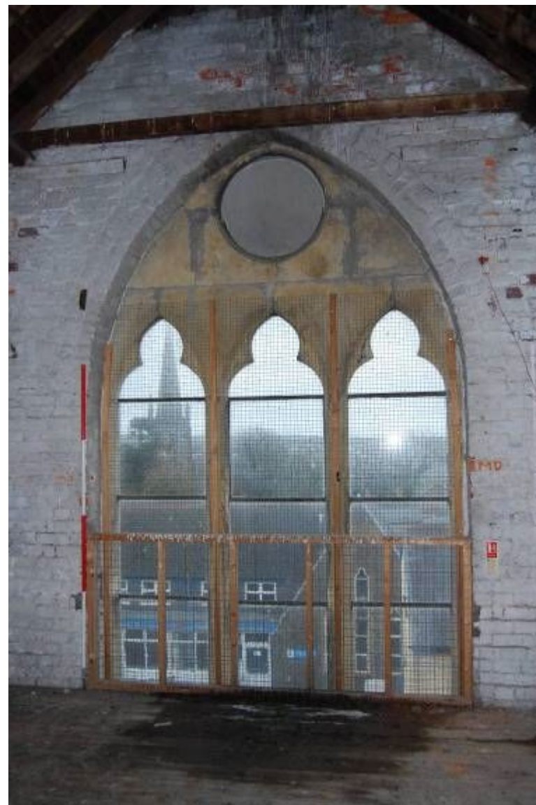
Plate 36. Second floor, east gable central window (from SW; 2m scale)
