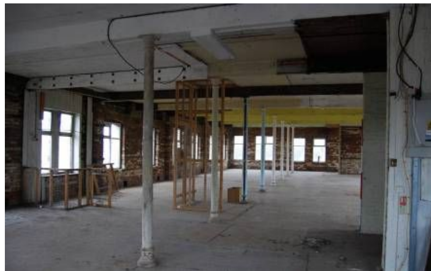
Plate 25. First floor (from WSW; 2m scale)
