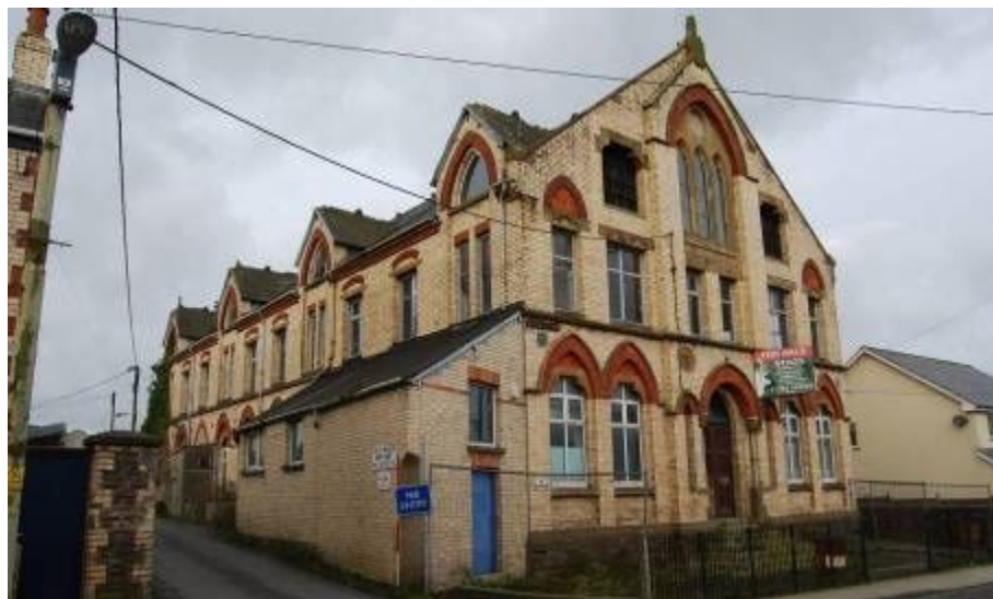
Plate 1. The Site exterior (from SE; 2m scale)
