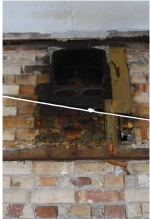
Plate 38. Heat vent, Area 3 (from ENE; Figure 4 )
