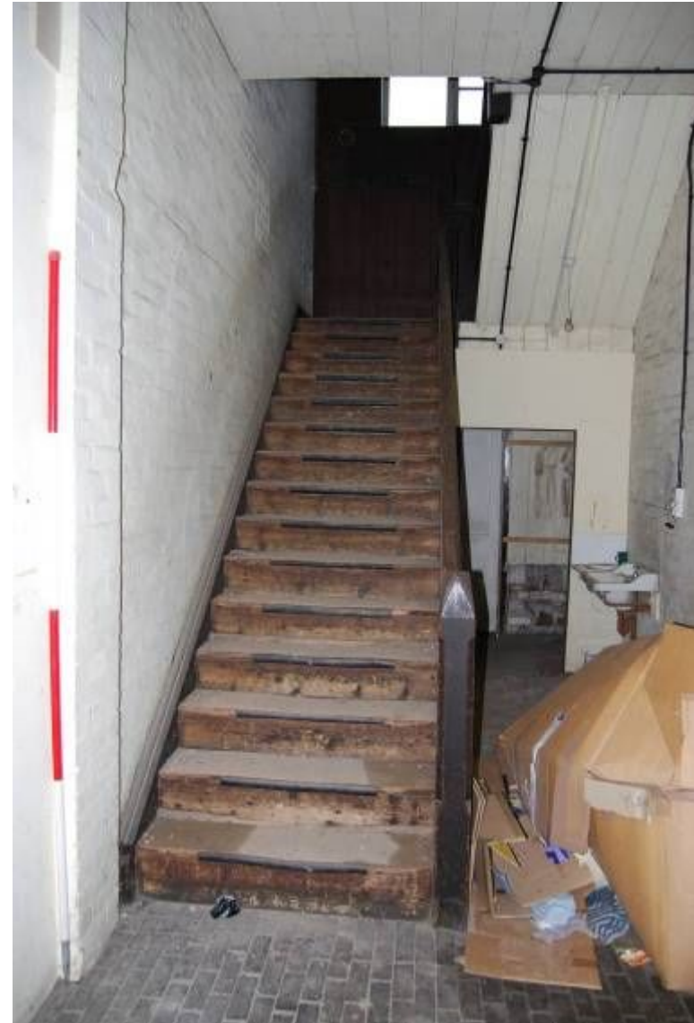
Plate 23. Area 5, staircase and brick floor (from NNW; 2m scale)
