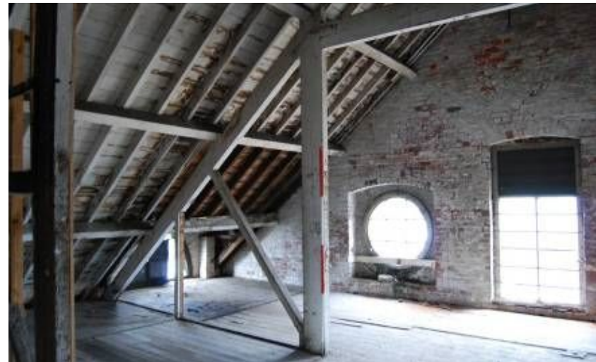
Plate 33. Second floor (from NE; 2m scale)
