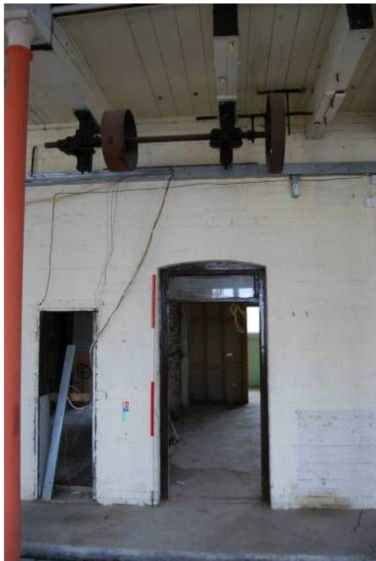
Plate 15. Area 4, access, Area 7 belt wheels (from NNW; 2m scale)
