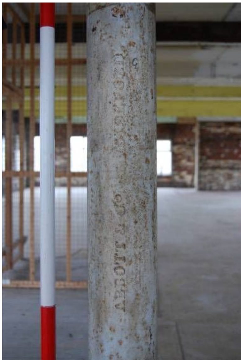
Plate 29. First floor, column detail (from SW; part 2m scale)
