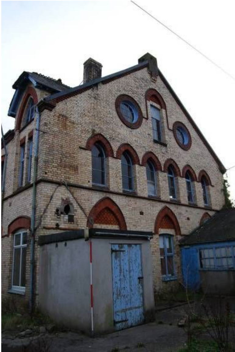
Plate 4. The Site exterior (from NW; 2m scale)
