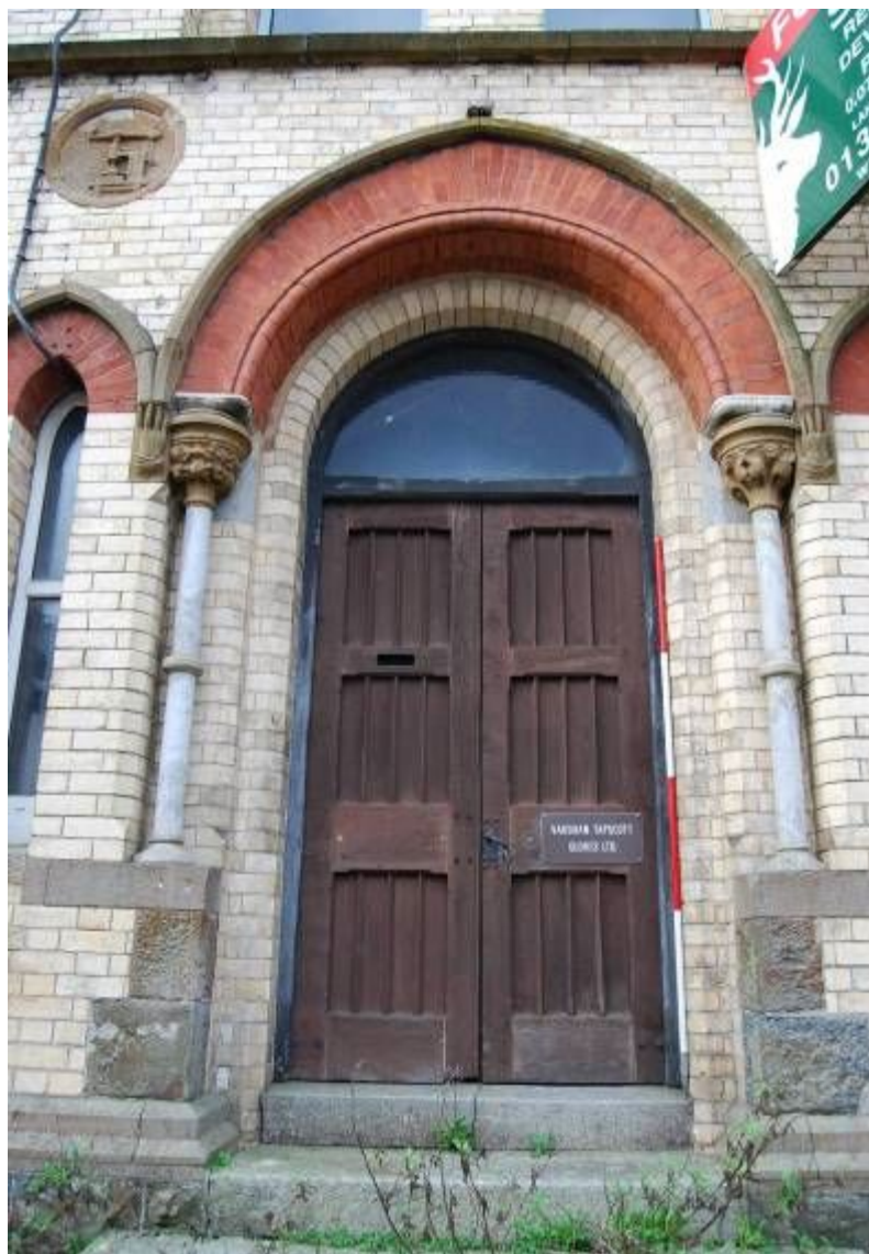
Plate 9. The Site exterior, front entrance (from ENE; 2m scale)
