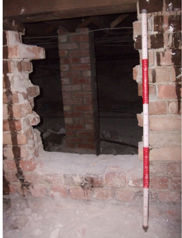
Plate 3. View into room B7 (from W; 1m scale)
