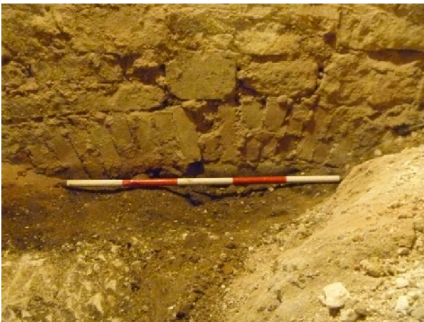
Plate 4. Underpinning (102) (from S; 1m scale)
