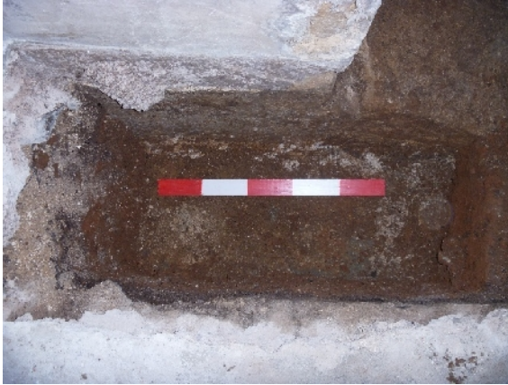
Plate 7. Tr4, threshold (403) of outshot door with white mortar (402) capping drain (from N; 0.5m scales)
