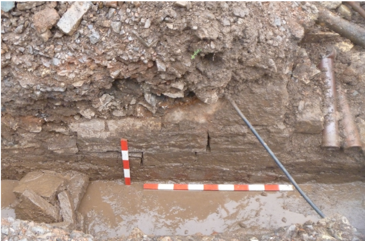
Plate 20. Tr10, east wall of culvert with large blocks of stone (1029) (from W; 0.50m & 1m scales)
