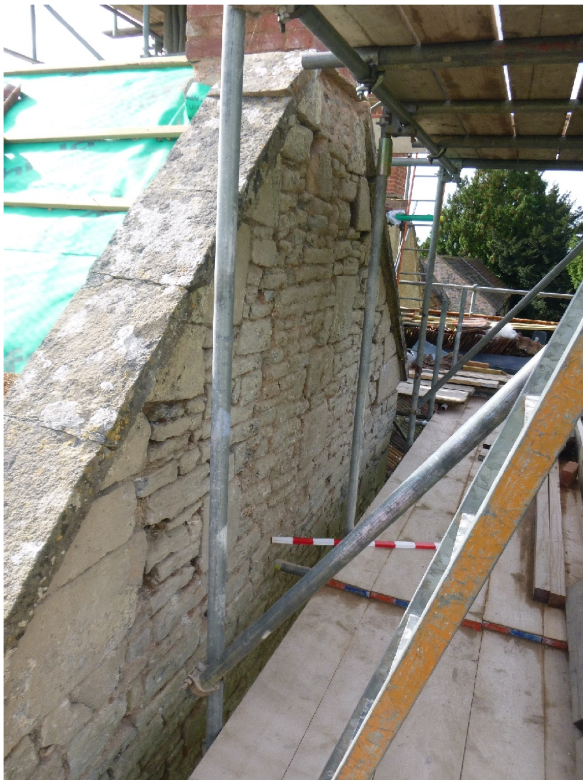
Plate 34. North gable wall of east range with re-use stones (from NEE; 1m scales)
