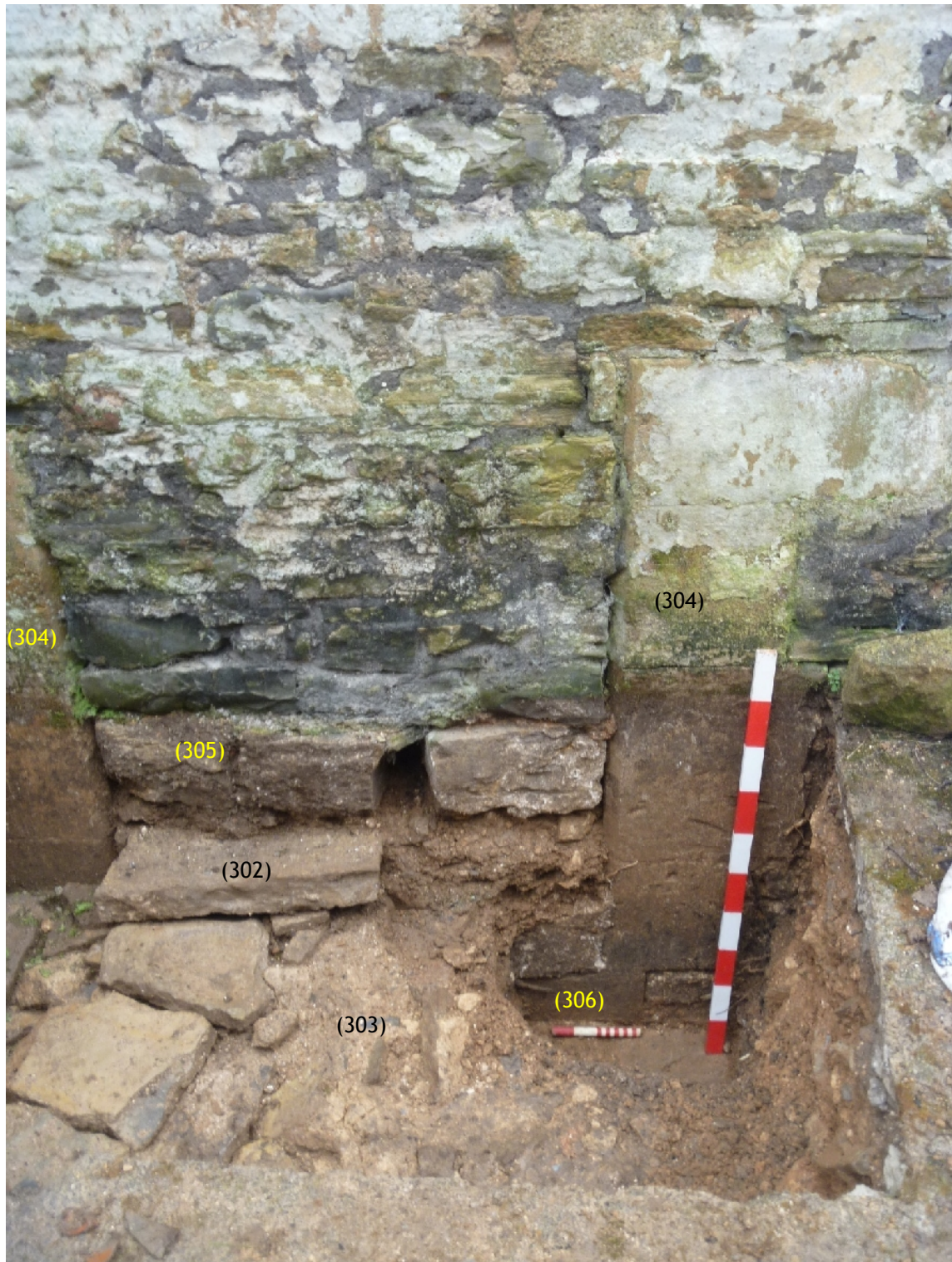
Plate 6. Tr3, blocked opening with aperture and drain (from N; 0.2m & 1m scales)
