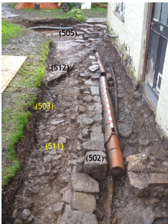
Plate 9. Tr5, modern drainage features and culvert (502) (from N; 1m scales)
