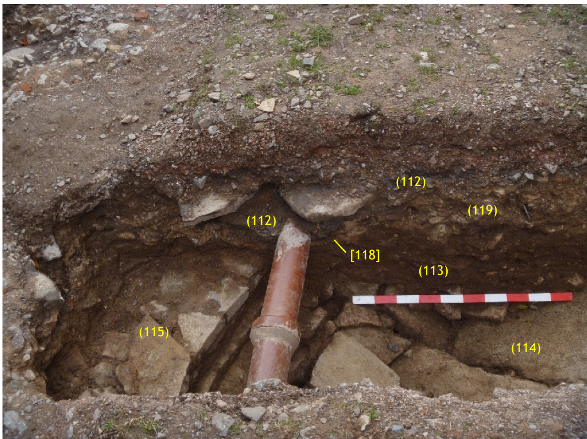
Plate 4. Tr1, paving (114) and wall (115) (from N; 1m scales)
