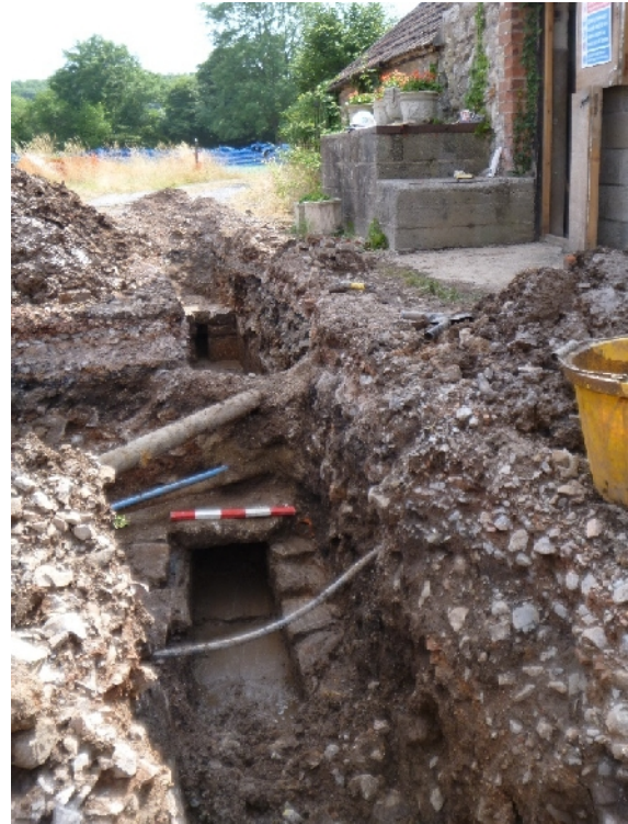
Plate 18. Tr10, culvert (1015) with dairy to west (from N; 0.5m scales)
