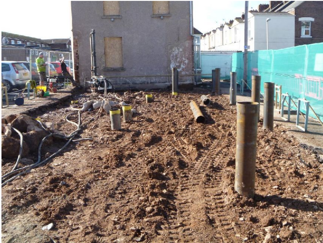
Plate 1. Pile trench 18 (from S; 1m scale)
