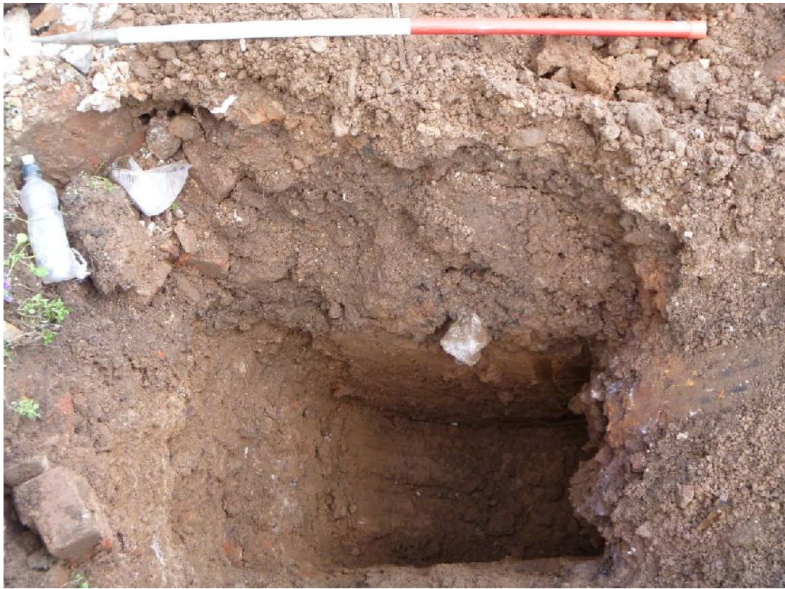
Plate 4. Pile trench 2 (from N; 1m scale)
