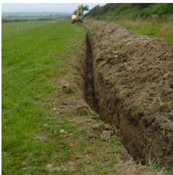
Plate 3. North pipe trench (from E; no scale)
