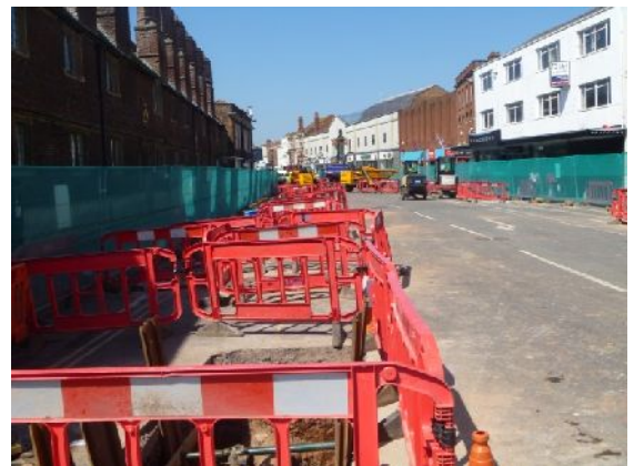
Plate 9. General works along East Reach, Pit 71 in foreground (from E)
