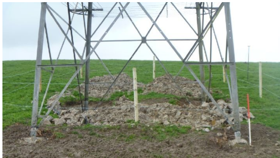
Plate 1: Tower YA30 after excavation of the bases (1m scale)
