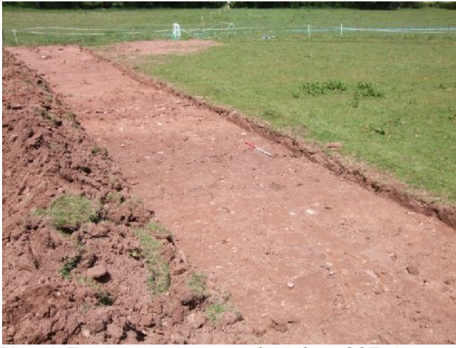
Plate 1. Easement strip across field (from SSE; 1m scale)
