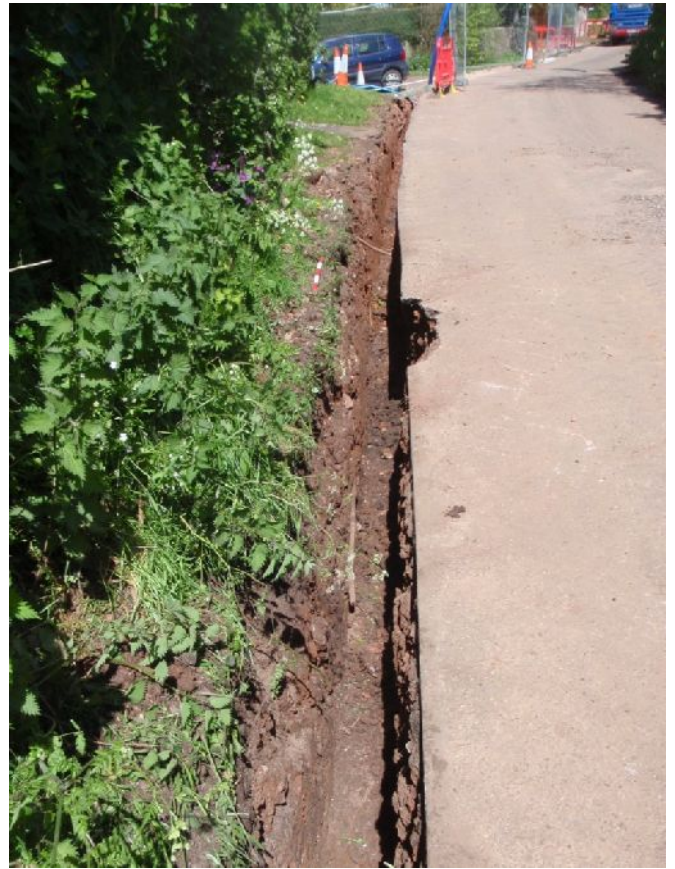
Plate 4. Road trench (from S; 1m scale)
