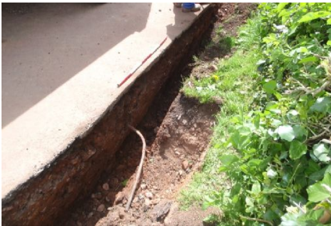
Plate 5. 19 th century water pipe (from E; 1m scale)
