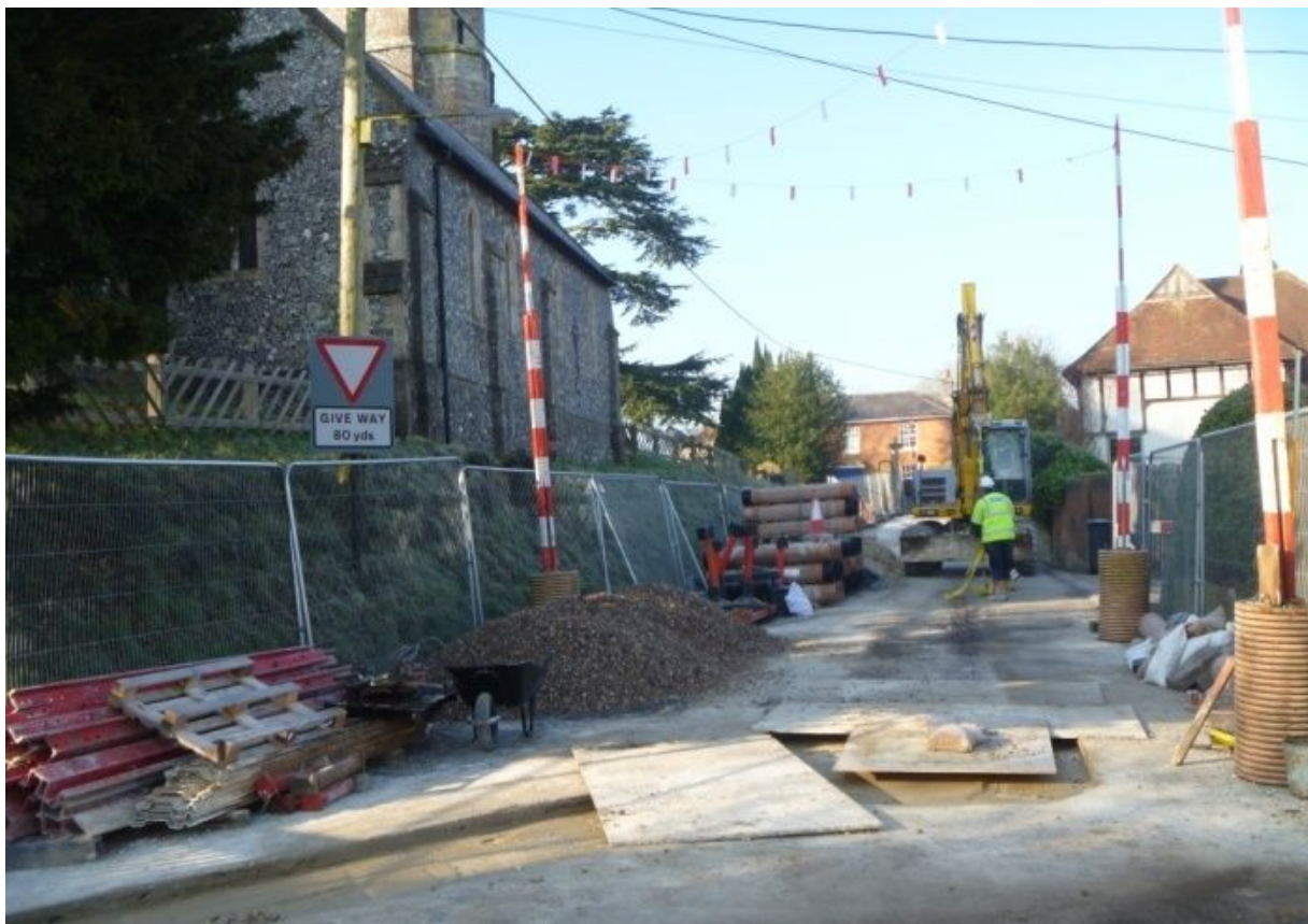
Plate 1. View of Church Street (from E end of pipeline route)
